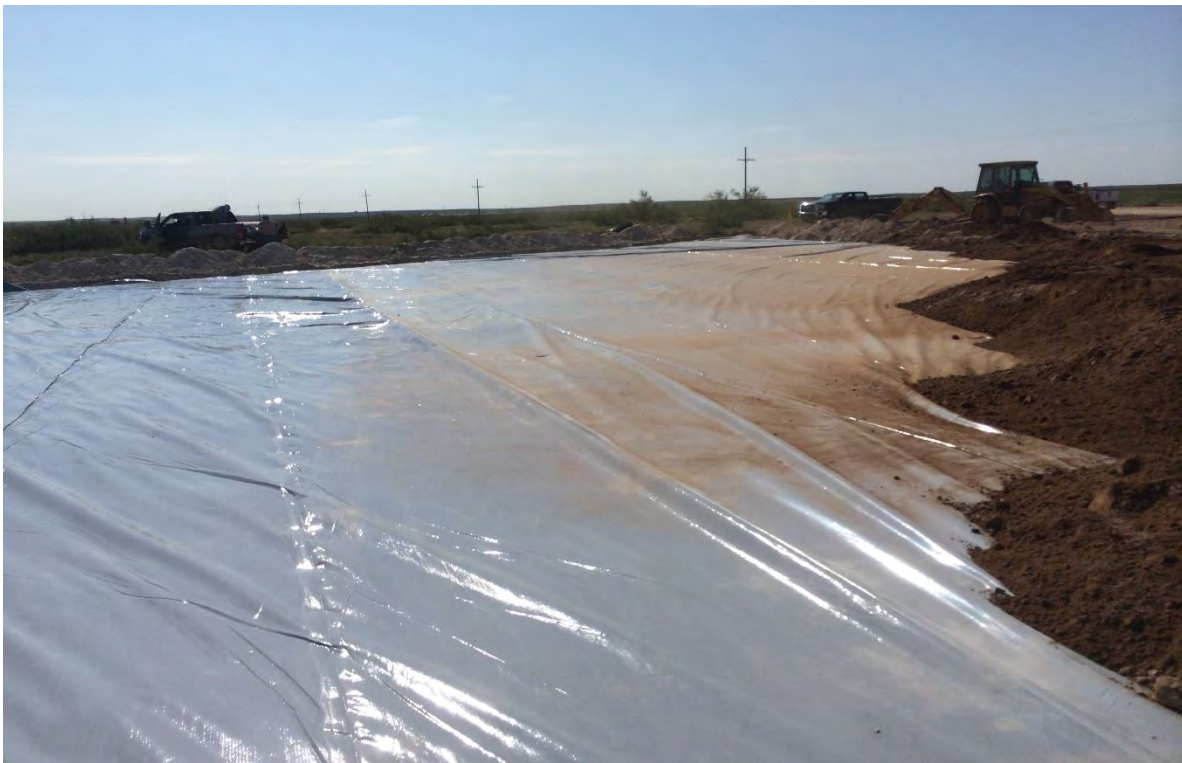
Indian Flats Bass Federal Well #3 - Liner Installation, Reserve Pit Area
