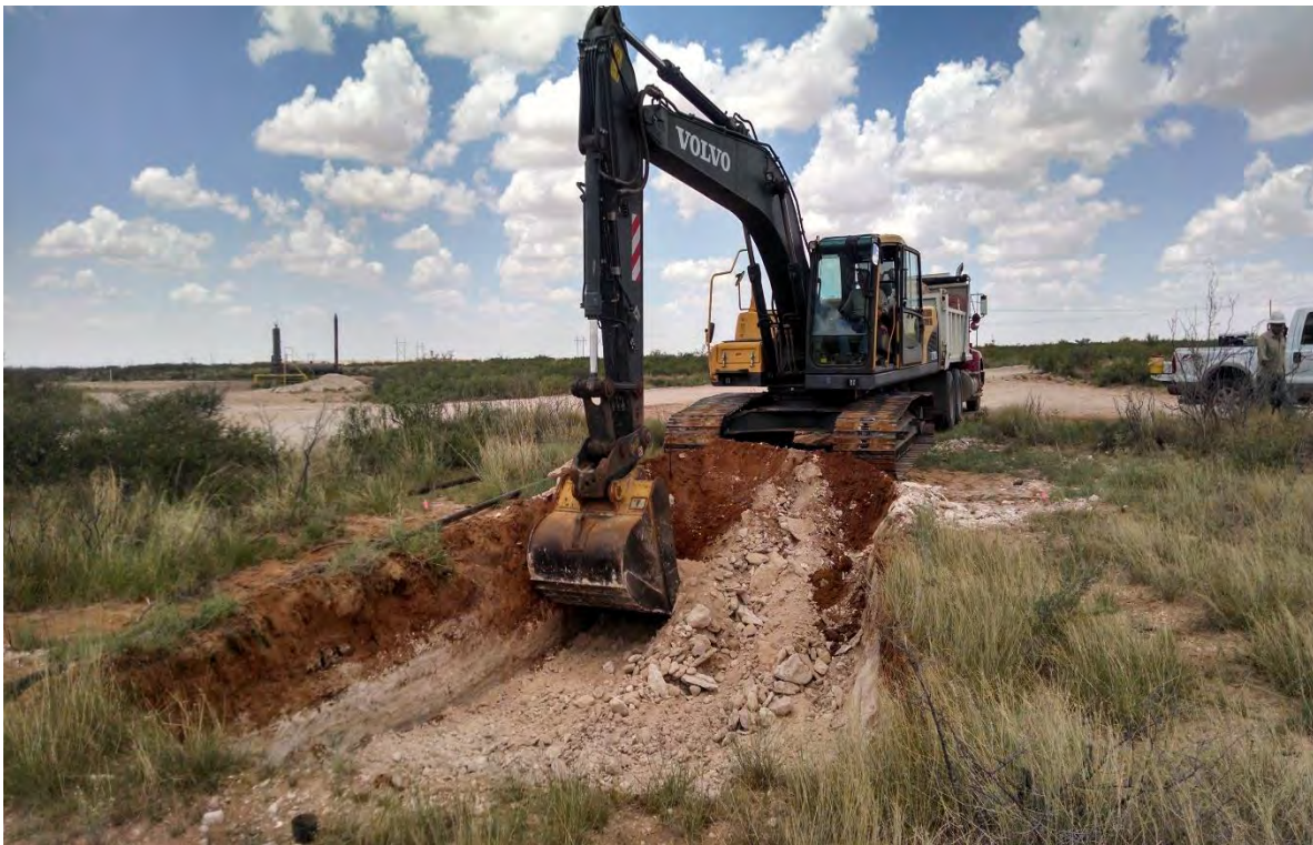
Golden “D” Federal Well #4 Flow Line – Pasture Excavation
