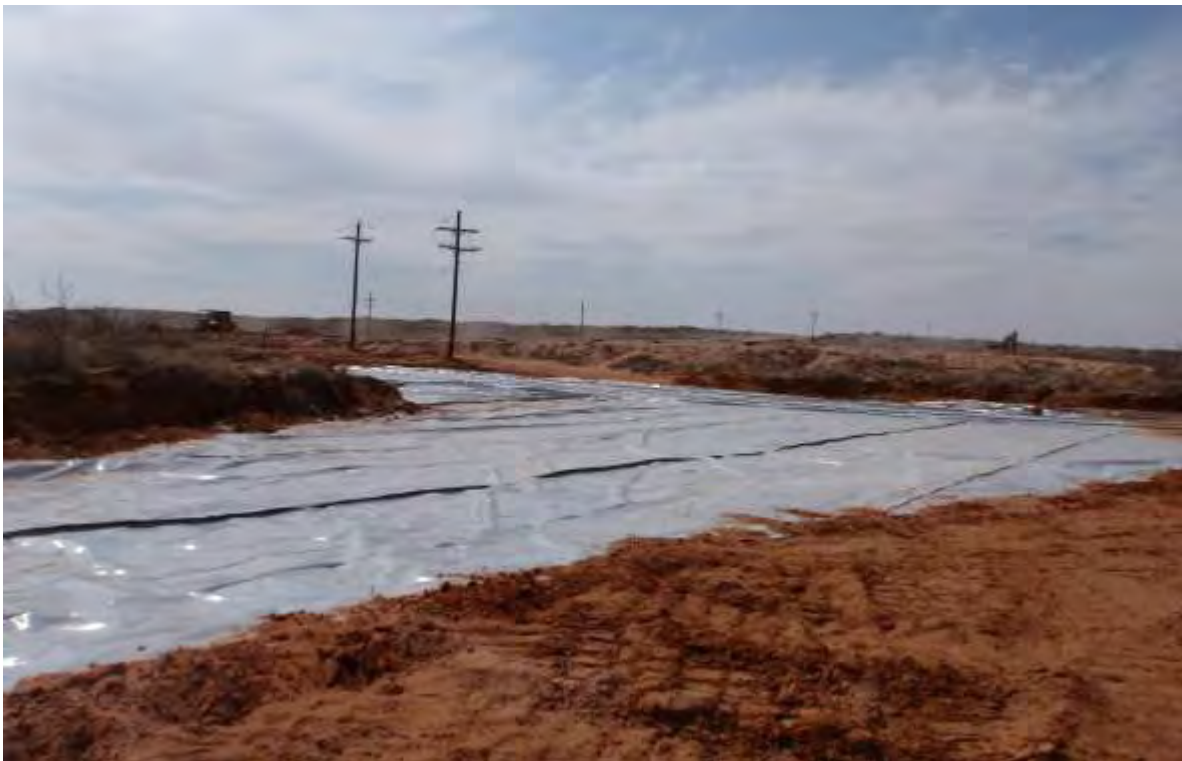
Poker Lake Unit #162 – Liner Installation
