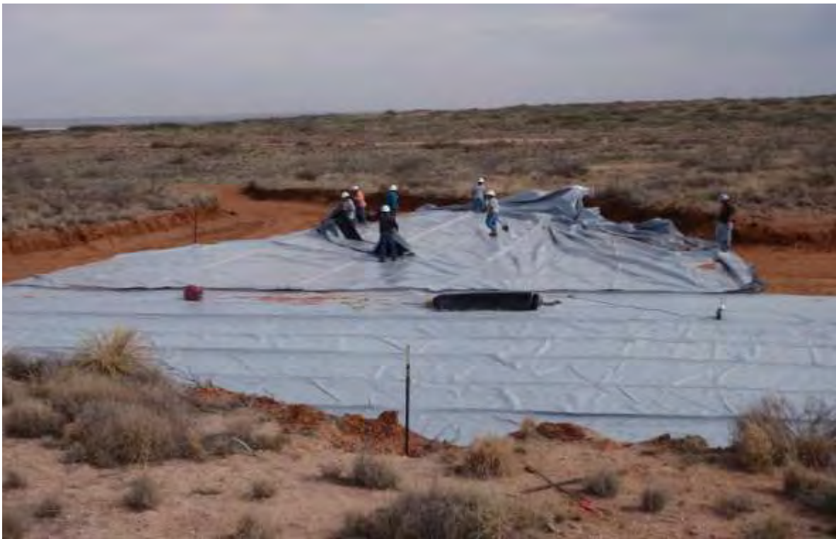
Poker Lake Unit #162 – Liner Installation
