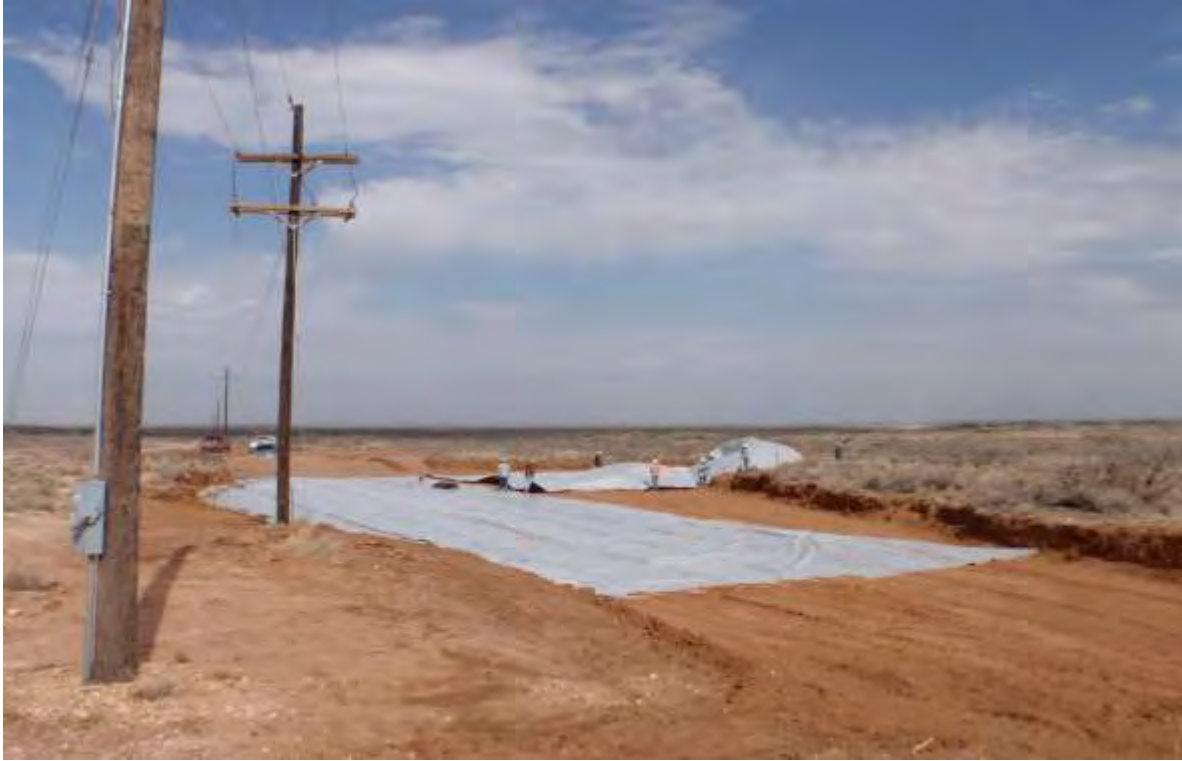
Poker Lake Unit #162 – Liner Installation
