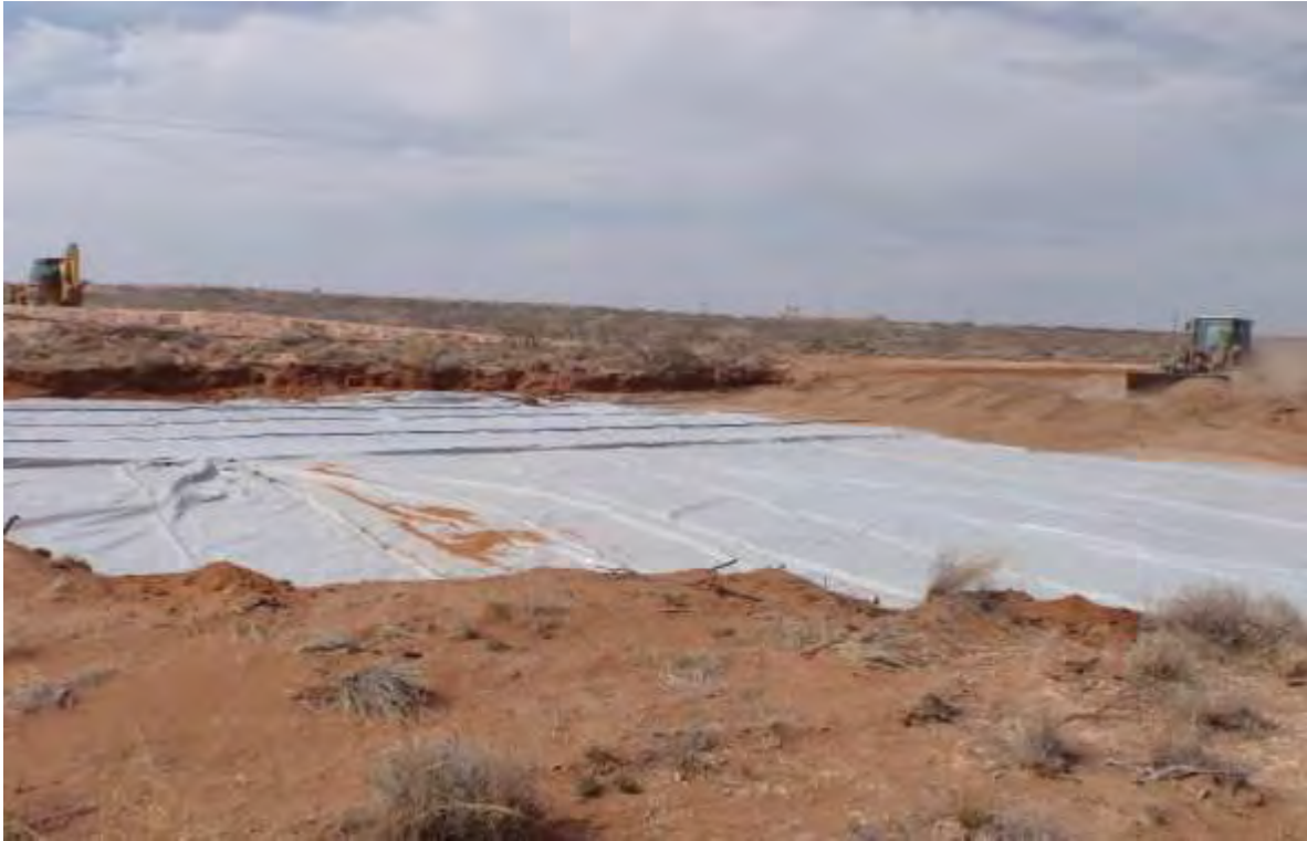
Poker Lake Unit #162 – Liner Installation & Backfilling
