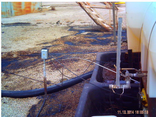
Oil Stain Inside Berm
