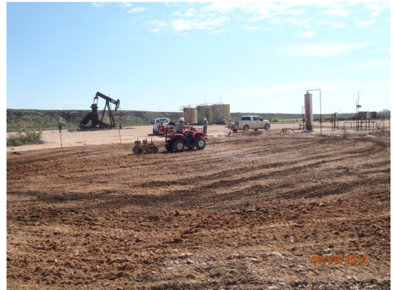
Disking amendments into soil, facing southeast 9/29/14
