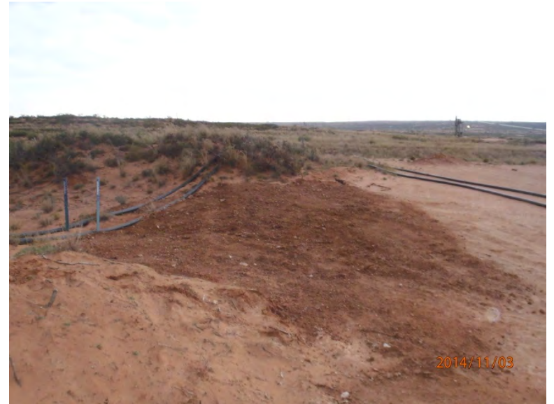
Site completed, facing east
