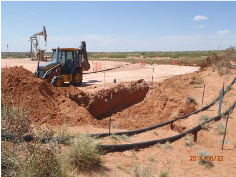
Excavation completed, facing southwest 8/22/14
