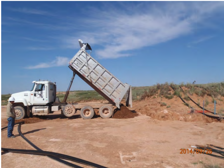
Importing soil, facing west 9/26/14
