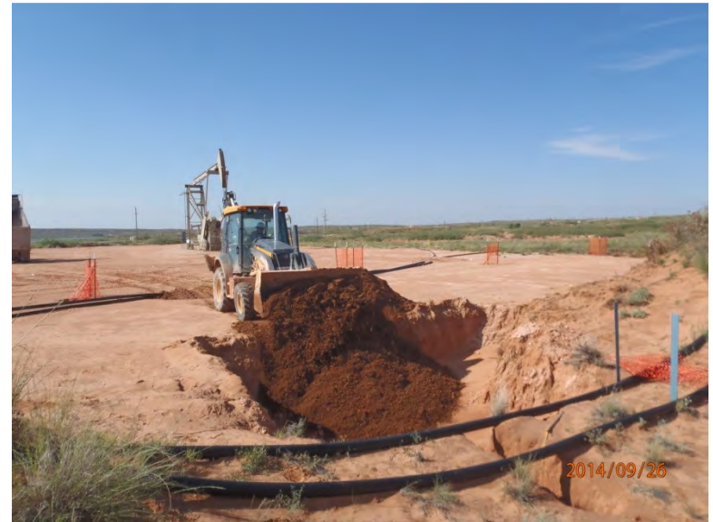
Backfilling site, facing south 9/26/14
