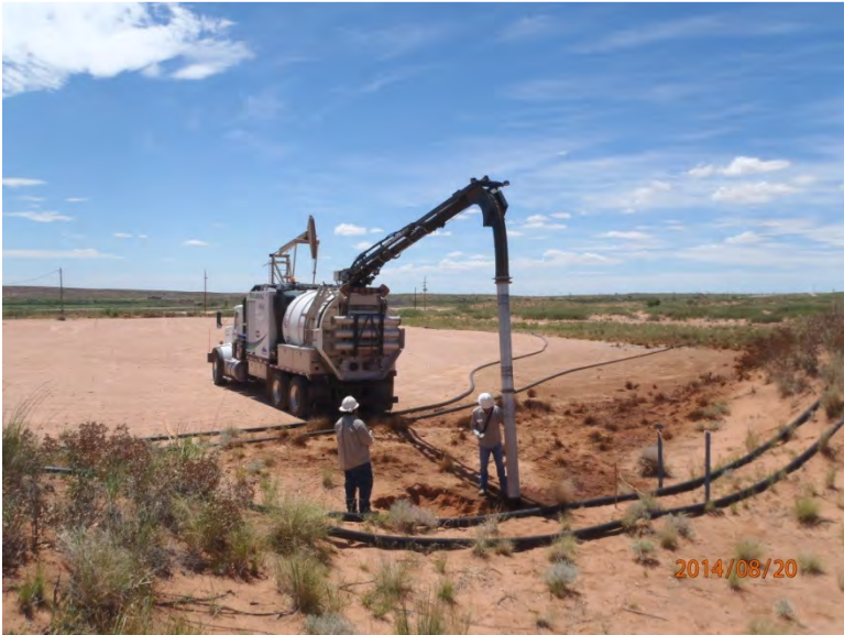
Excavating with hydro-vac, facing southwest 8/20/14
