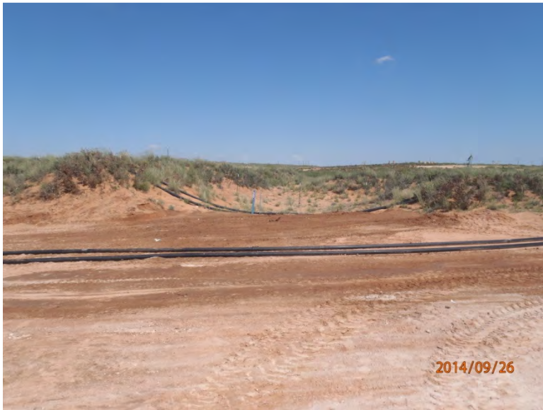
Site backfilled, facing north
