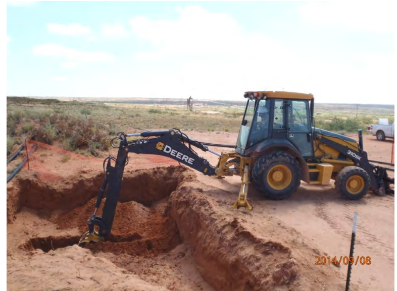
Installing vertical in base of excavation, facing east 9/8/14
