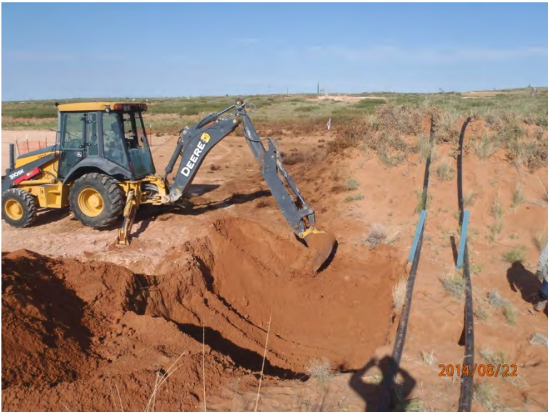
Excavating release area, facing west 8/22/14
