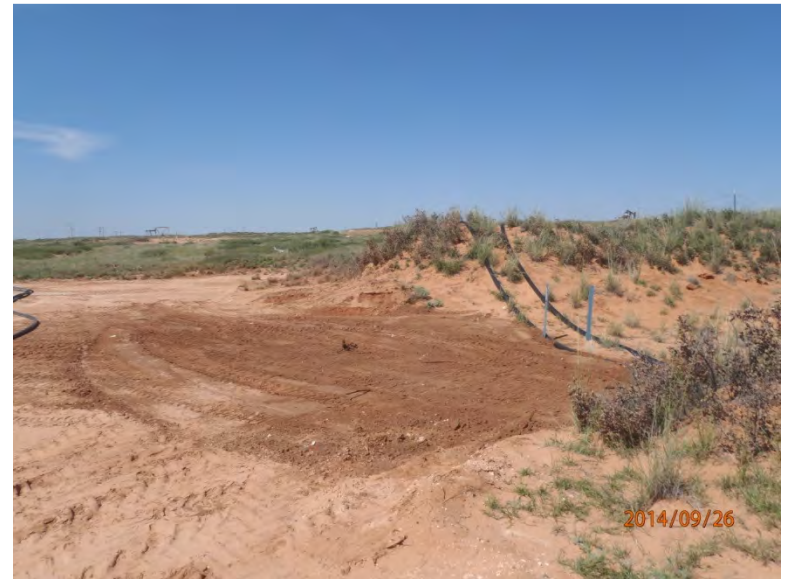
Site backfilled, facing west
