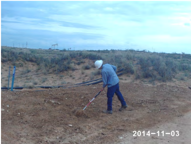
Raking site prior to seeding, facing northeast
