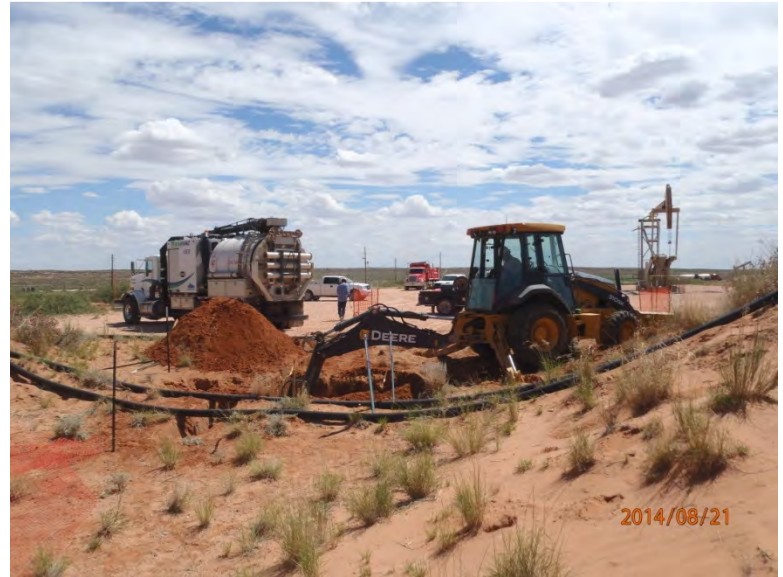
Installing vertical, facing south 8/21/14
