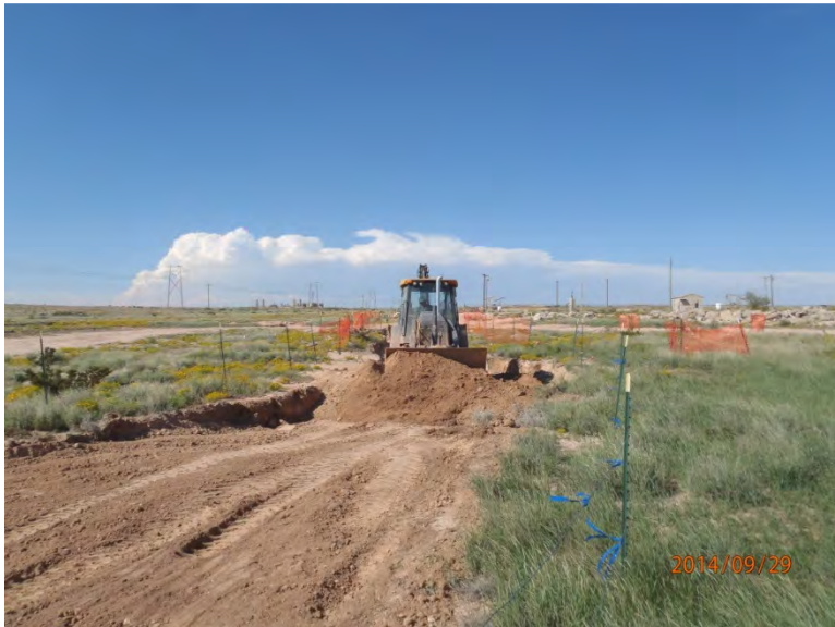
Backfilling excavations, facing north 9/29/14
