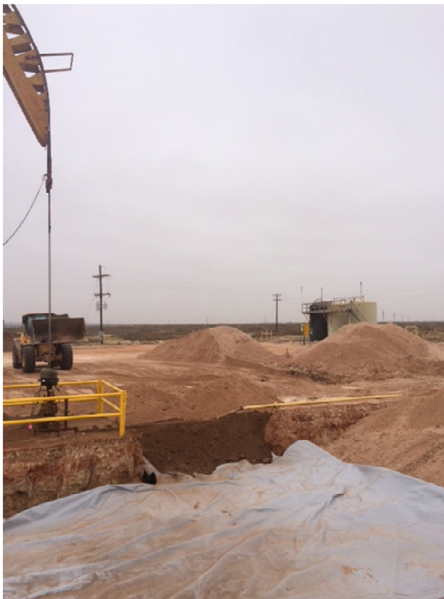
Photograph of the installed liner at the BEU #143 Remediate Site.
