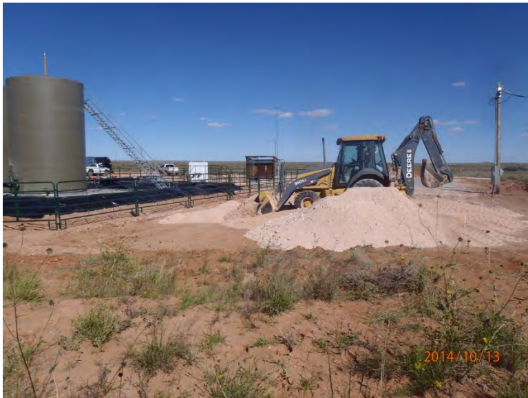
Backfilling 6 inch scrape on south side of facility, facing east 10/13/14
