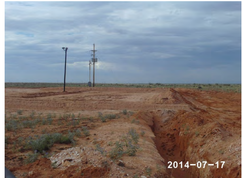
6 inch scrape on pad completed with berms installed, facing south 7/17/14
