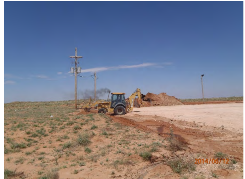
Scraping pasture area to 6 inches bgs, facing west
