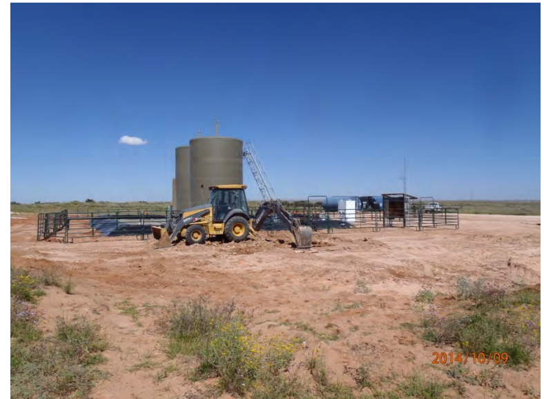
Beginning 6 inch scrape on south side of new facility, facing north 10/9/14
