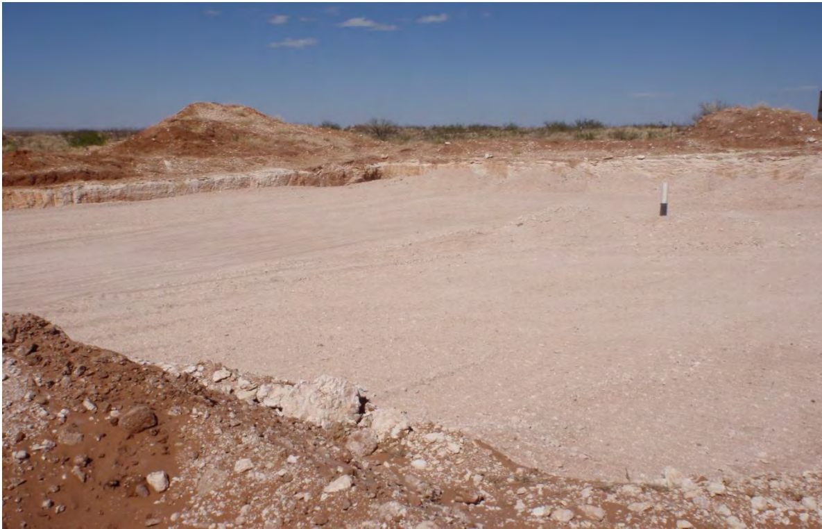
G.H. Cobb Federal #1 - Excavation (following liner installation and backfilling)
