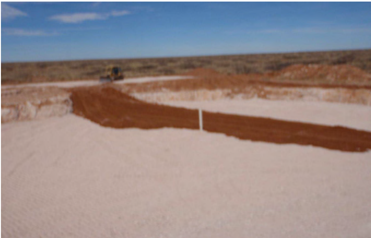
G.H. Cobb Federal #1 - Backfilling & Installation of Pad Sand
