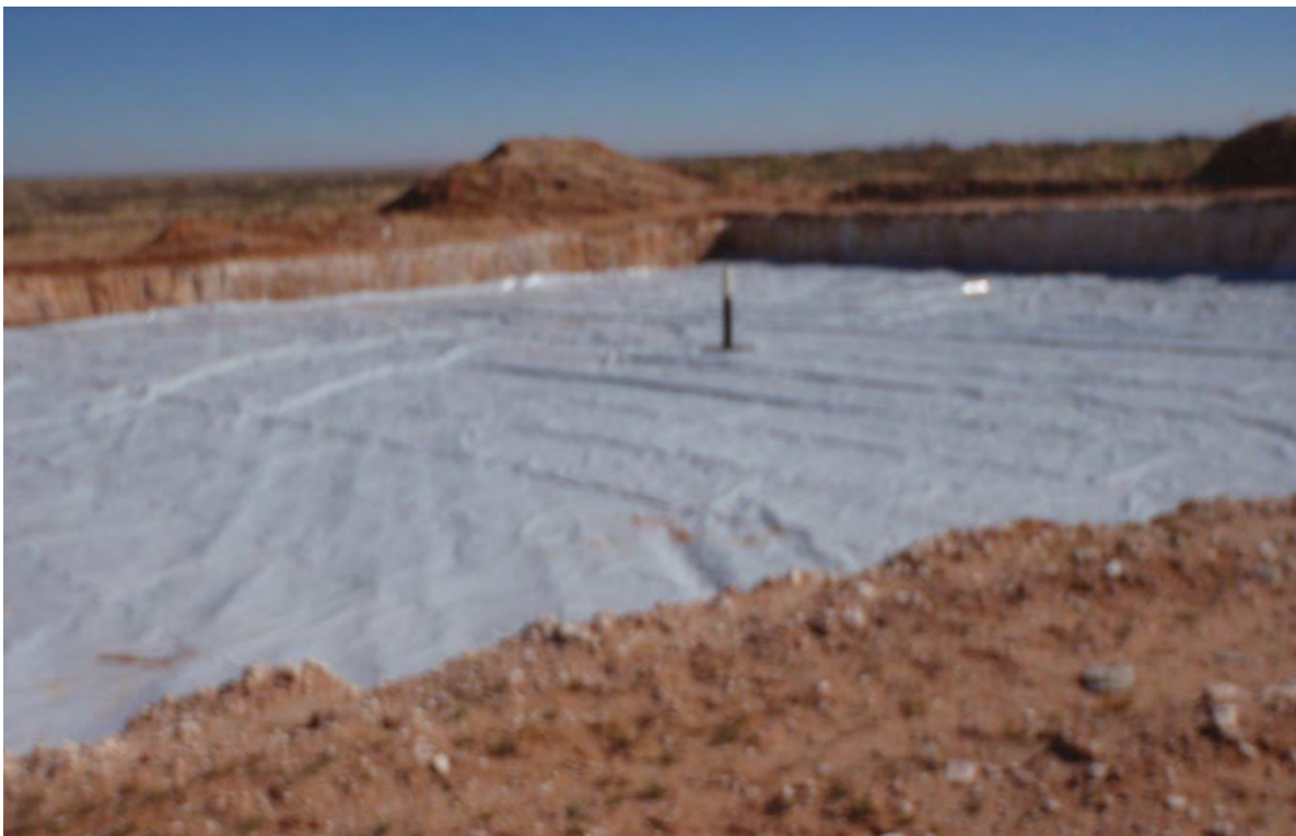
G.H. Cobb Federal #1 - Liner Installation
