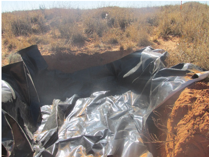
Installation of 20 mil liner 11/25/2014
