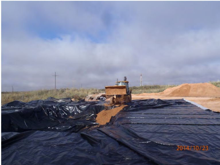
Direct burying contaminated soil from release, facing west 10/23/14
