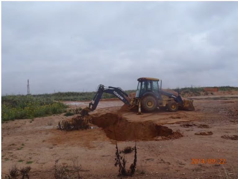
Excavating to 8 ft for direct bury, facing northwest 9/22/14
