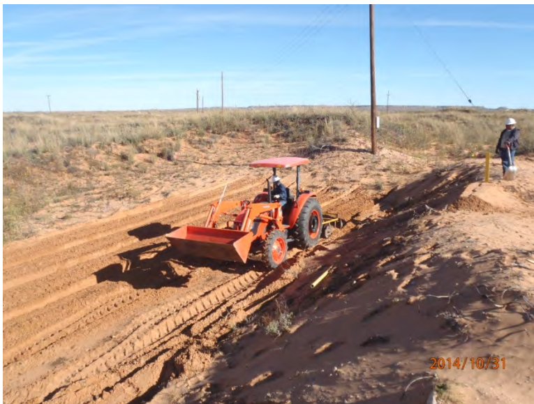
Disking in soil amendments over release area, facing northeast 10/31/14
