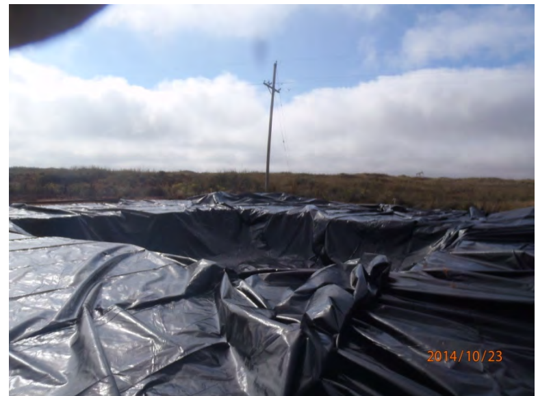
Installing 20-mil liner in 8 ft excavation, facing southeast 10/23/14
