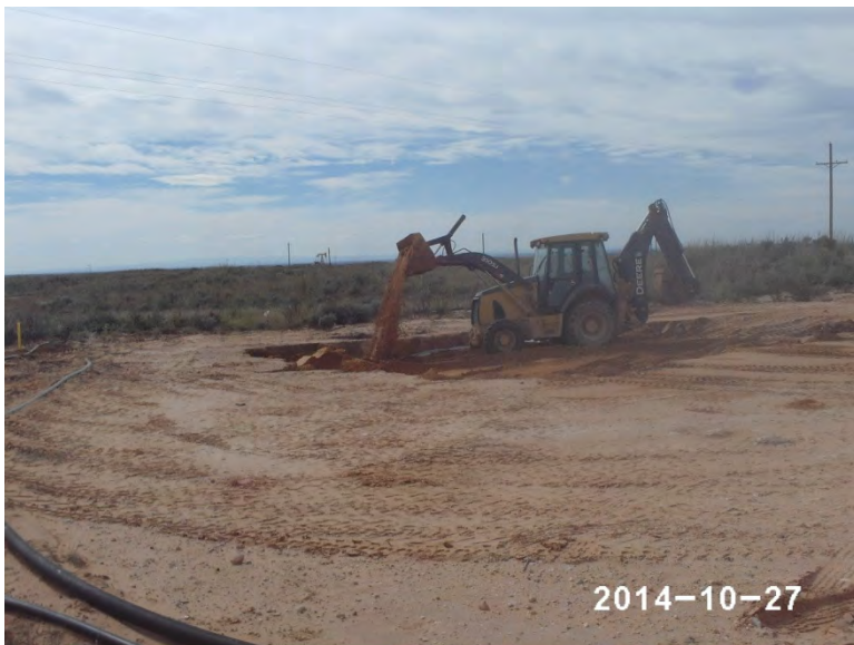
Backfilling direct bury with the removed caliche, facing southwest 10/27/14
