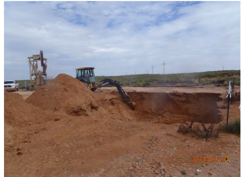
Continuing to excavate to 8 ft for direct bury, facing northeast 9/23/14
