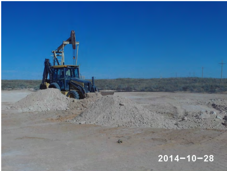
Backfilling direct bury with the imported caliche, facing northeast 10/28/14
