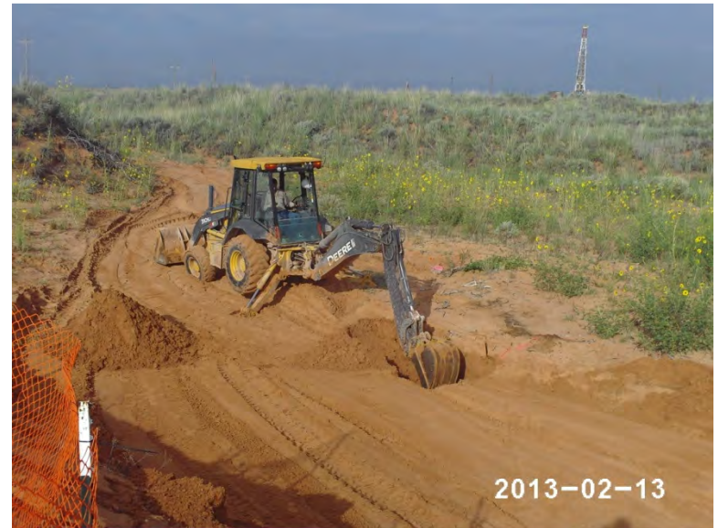
Excavating to 3 ft, facing southwest 9/17/14
