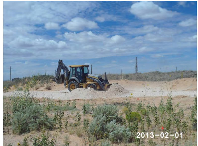
Constructing caliche road to facilitate excavation activities, facing southwest
