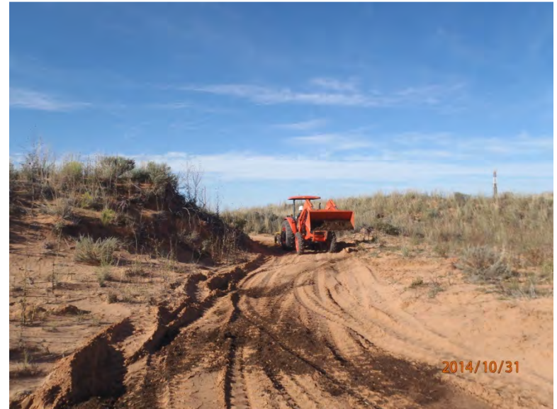
Spreading soil amendments over release area, facing west 10/31/14
