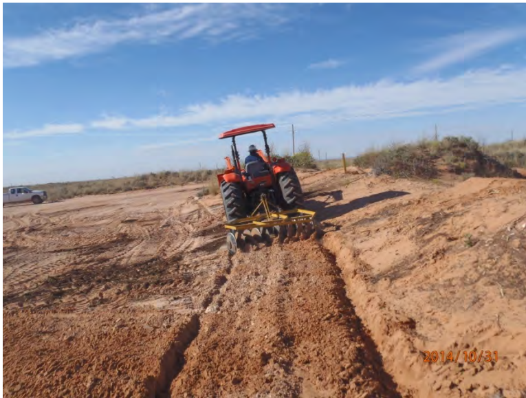
Disking soil amendments over direct bury area, facing west 10/31/14
