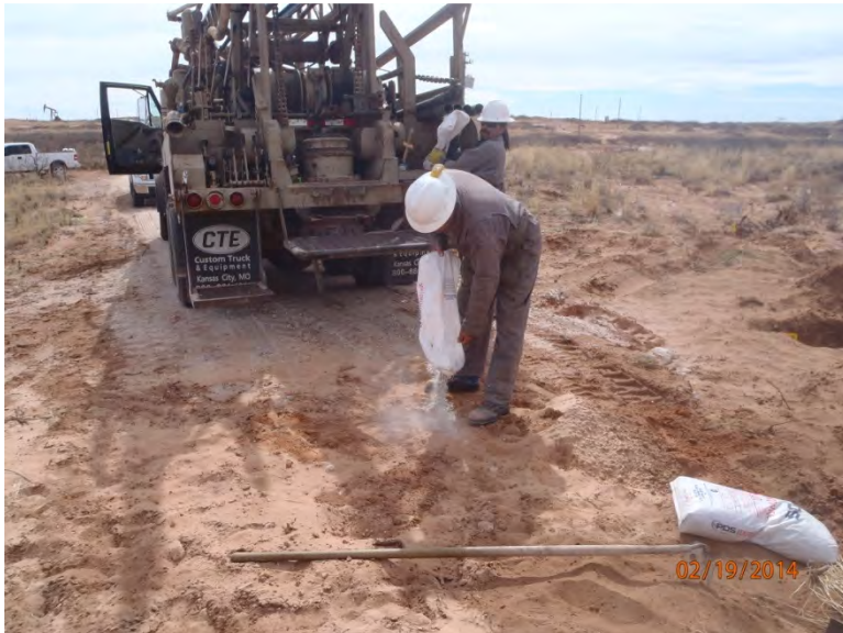
Plugging SB-3 in total with bentonite
