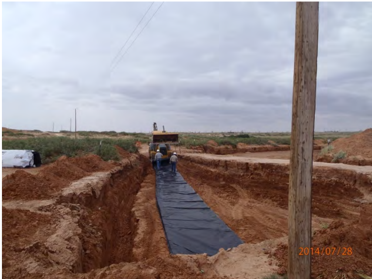
Installing 20-mil reinforced liner, facing south 7/28/14
