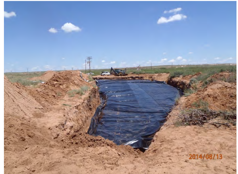
Liner installation completed, facing east
