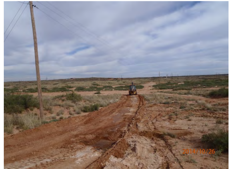
Scraping up caliche road, facing north
