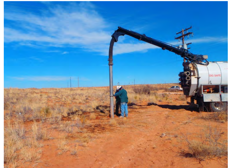
Line spot with hydrovac, facing north 1/28/14
