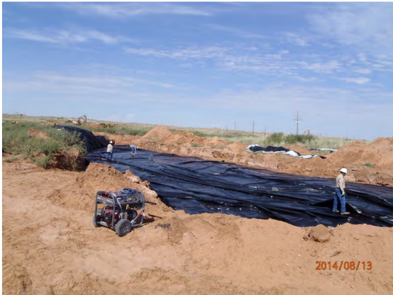
Installing 20-mil reinforced liner, facing west
