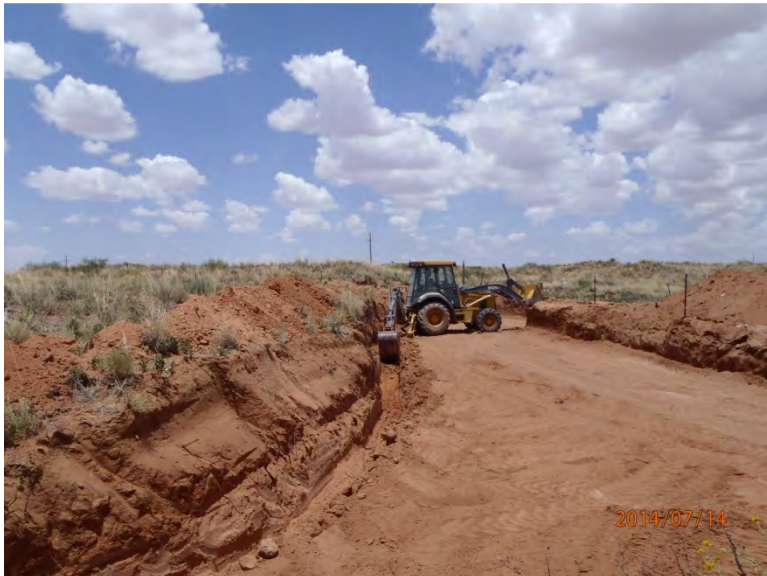
Digging trench to keyset liner, facing northwest 7/14/14
