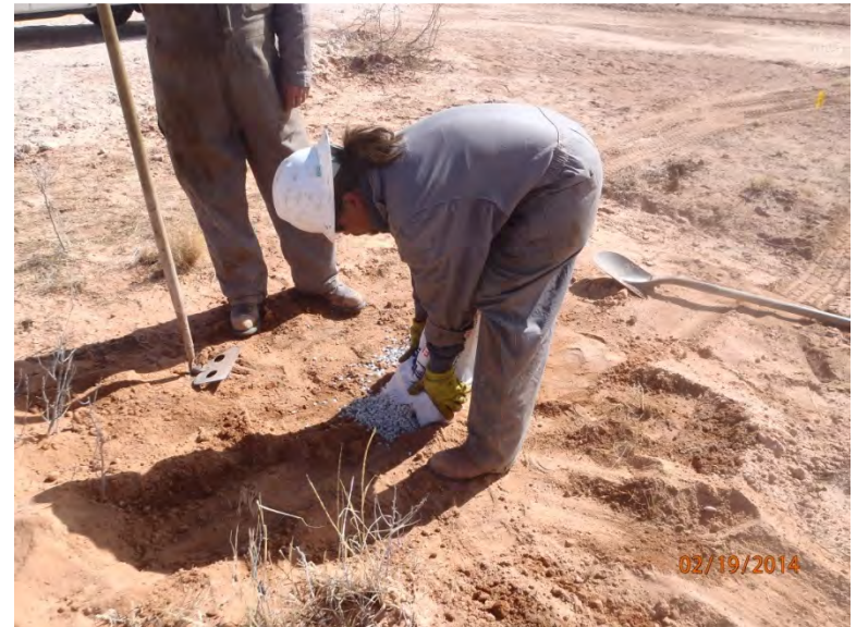
Plugging SB-2 in total with bentonite 2/19/14
