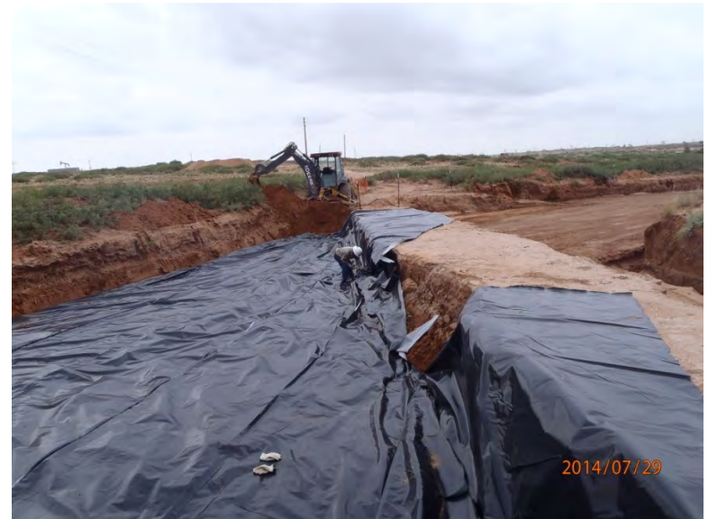
Installing 20-mil reinforced liner, facing south 7/29/14
