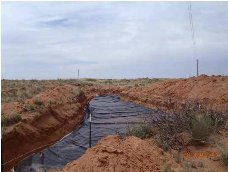
Liner installation completed, facing northwest 7/29/14
