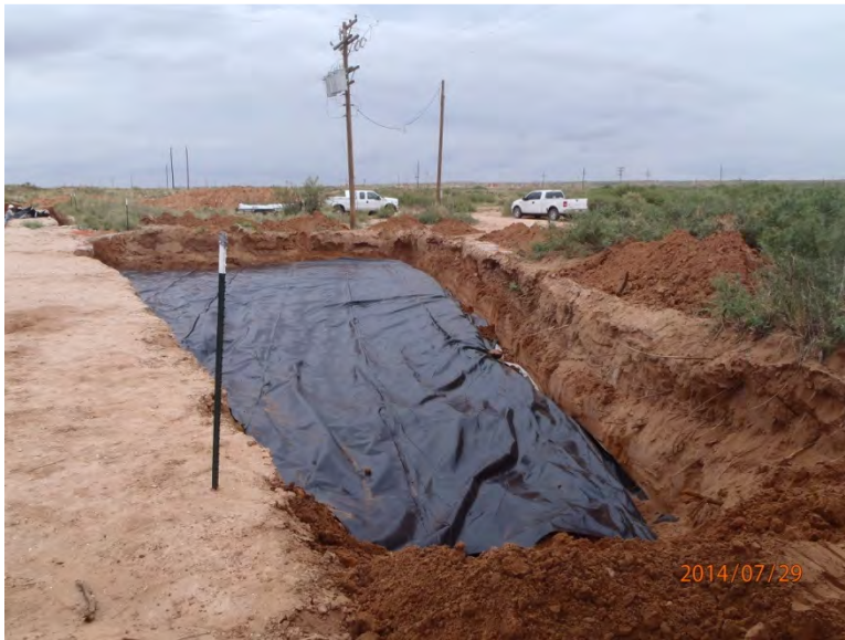
Liner installation completed, facing northeast 7/29/14
