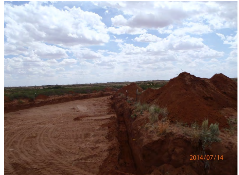
Trench for keyset completed, facing southwest 7/14/14
