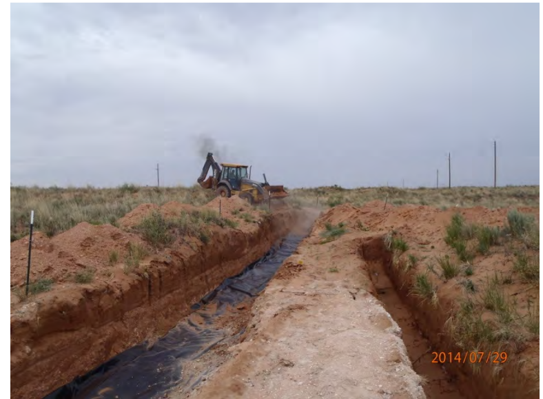
Liner installation completed, facing north 7/29/14
