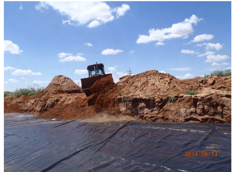
Key-setting liner, facing northwest 8/13/14
