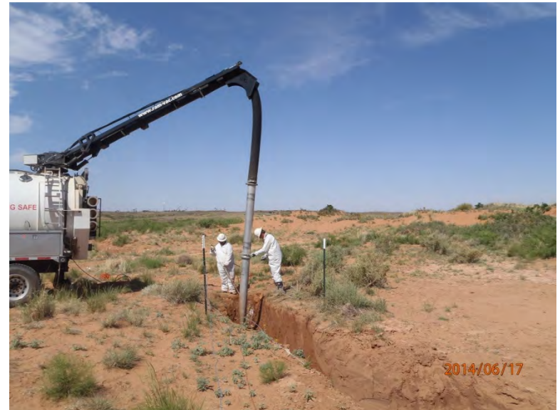
Hydro-excavating around buried lines, facing southwest 6/17/14
