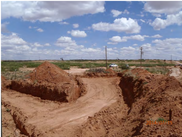
Trench for keyset completed, facing northeast 7/15/14
