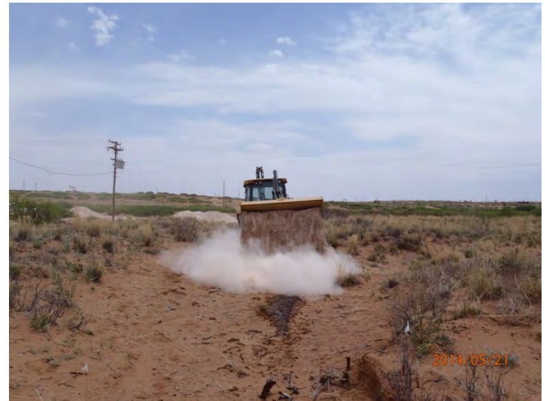
Construction caliche road to site to facility excavation activities, facing south 5/21/14
