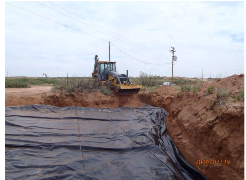
Key-setting liner, facing southeast 7/29/14
