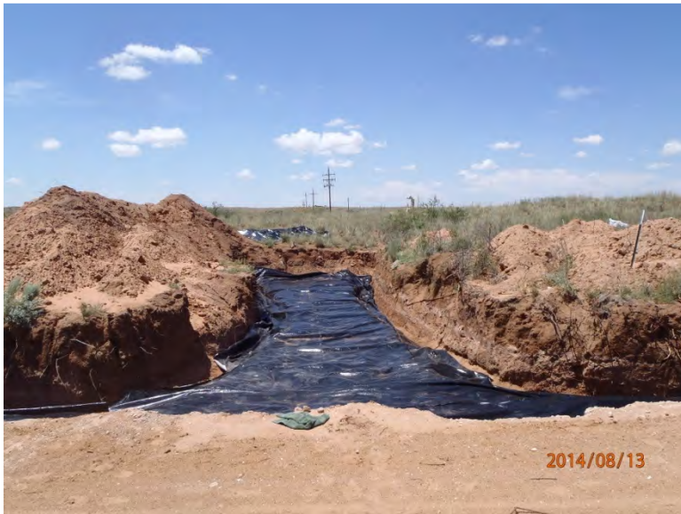
Liner installation completed, facing west 8/13/14
