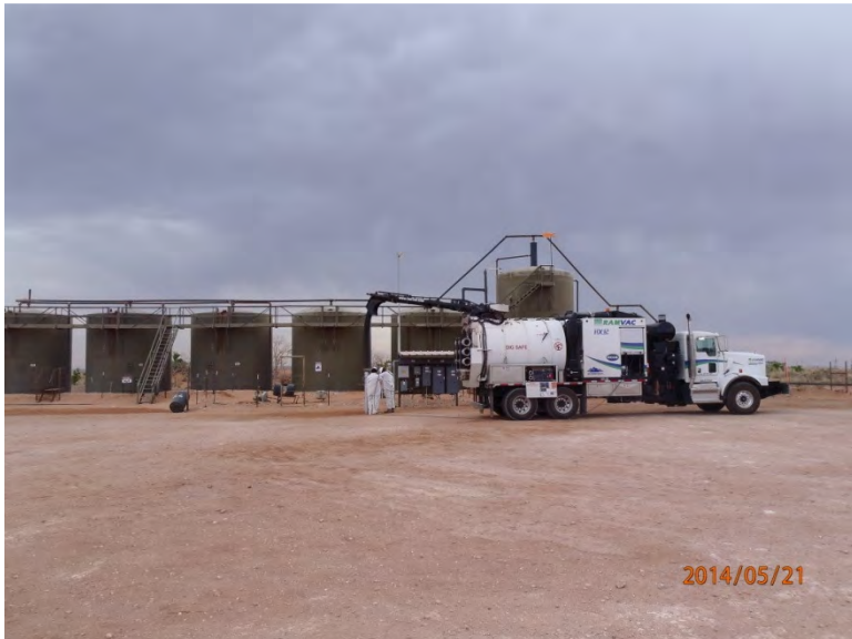
Using hydro-vac to line spot, facing north 5/21/14
