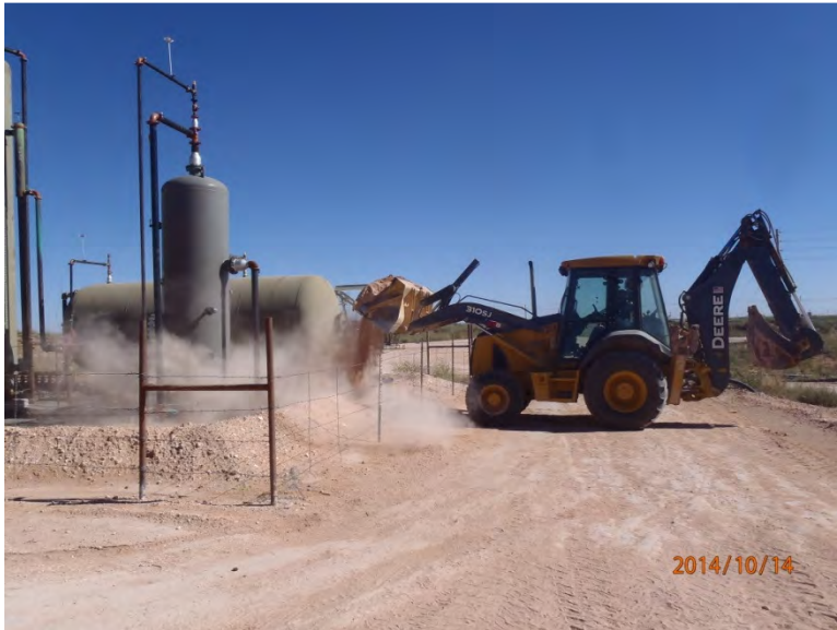
Installing berms, facing northeast
