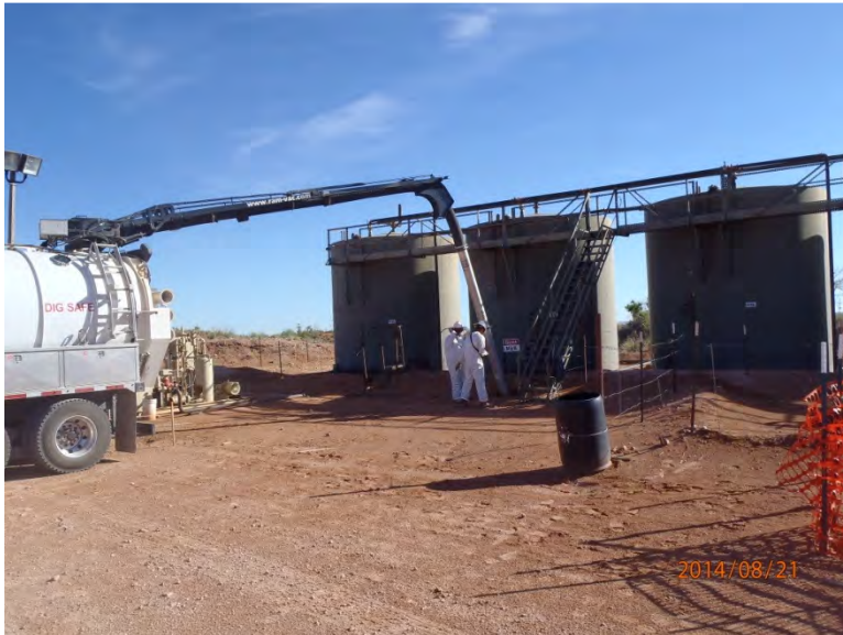
Hydro-excavating near tanks, facing northwest 8/23/14
