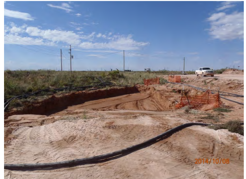
Excavation to 3 ft completed, facing west
