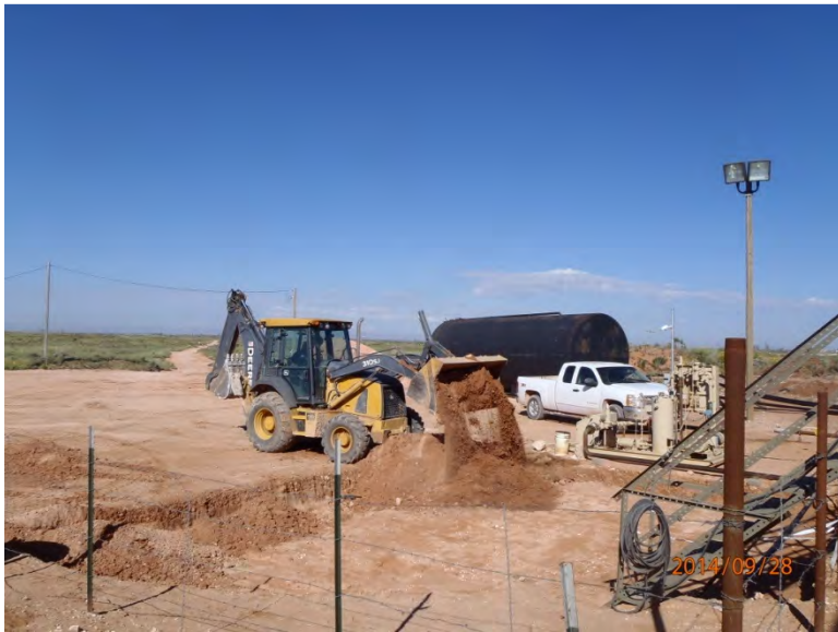
Backfilling hydro-excavation, facing northwest 9/28/14
