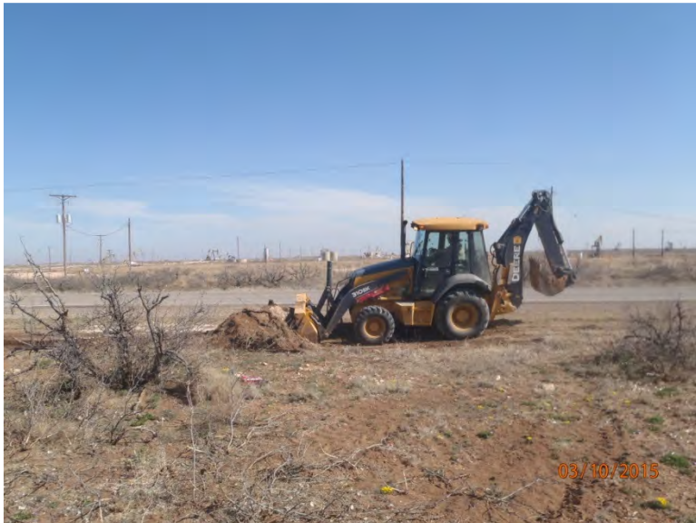
Scraping bar ditch, facing north
