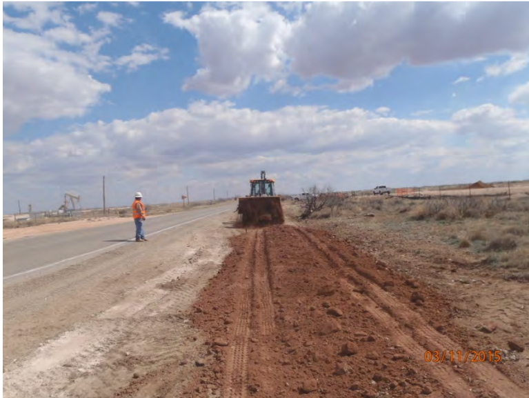
Backfilling release with imported soil, facing east 3/11/15
