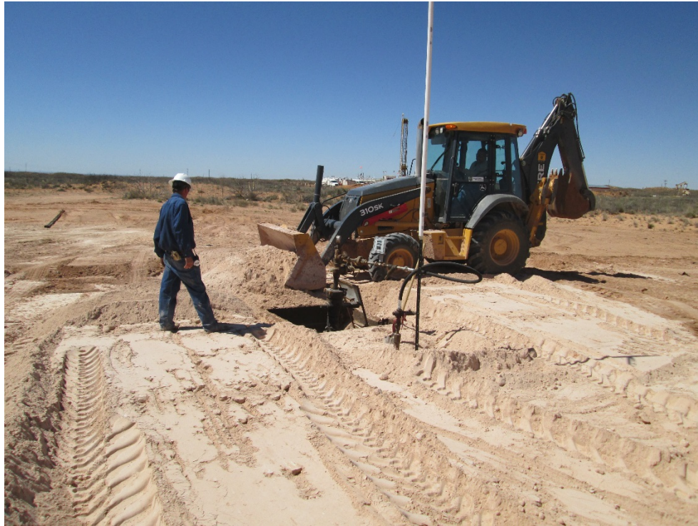
Backfilling pad with fresh caliche
