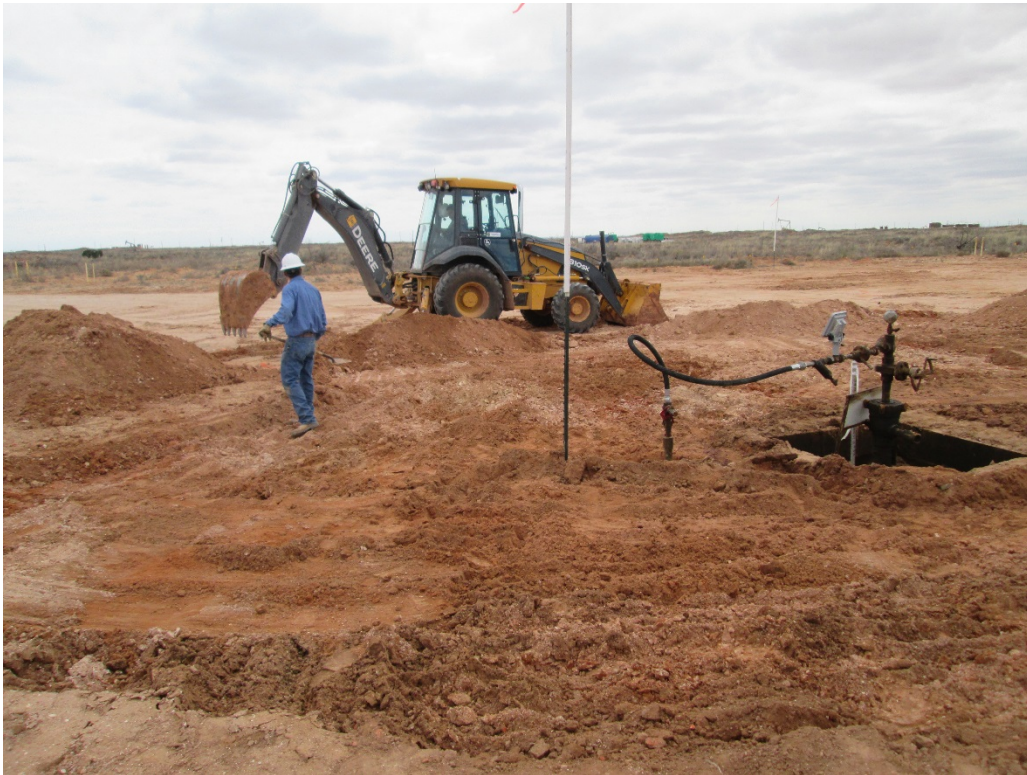
Excavating area around injection well on pad
