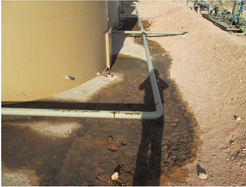
PHOTO 1: VIEW FACING WEST OF THE TANK BATTERY SHOWING PRODUCT SATURATED SOIL ALONG THREE CRUDE OIL TANKS
