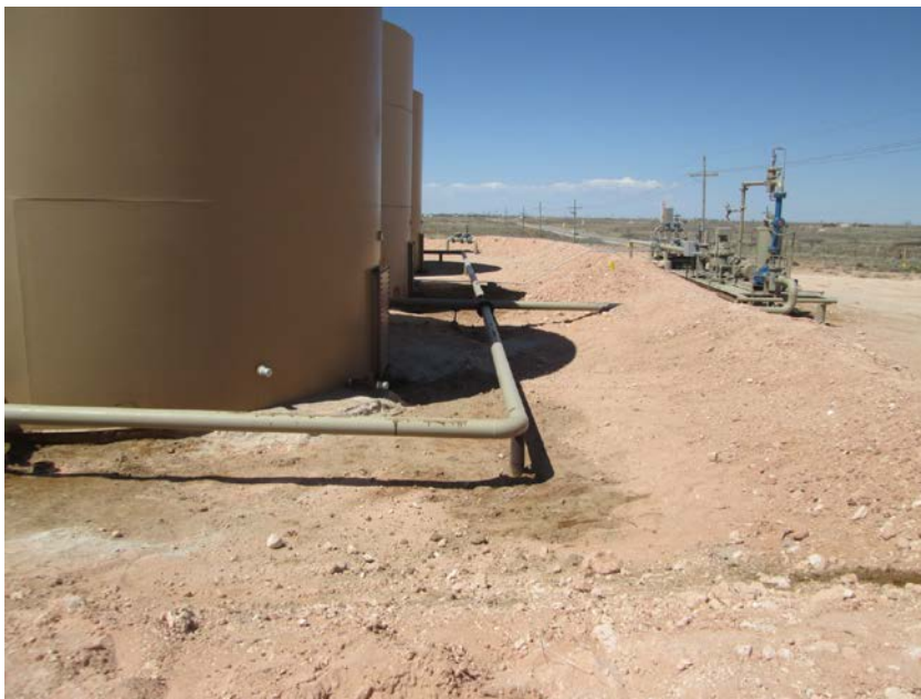
PHOTO 5: VIEW FACING WEST OF THE TANK BATTERY SHOWING REMEDIATED SOIL ALONG THREE CRUDE OIL TANKS
