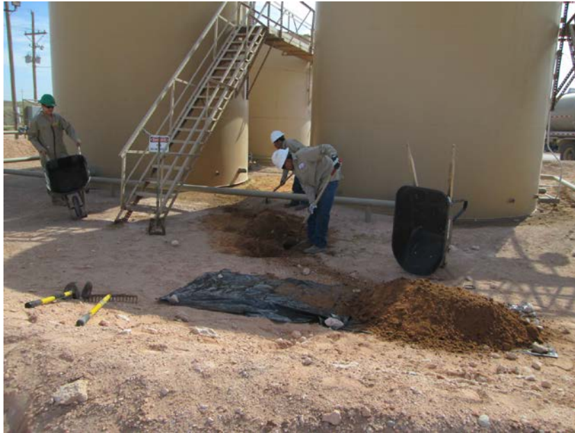
PHOTO 3: VIEW FACING NORTH EAST OF THE TANK BATTERY SHOWING SEVERAL LOBO'S CREW MEMBERS REMOVING PRODUCT SATURATED SOIL
