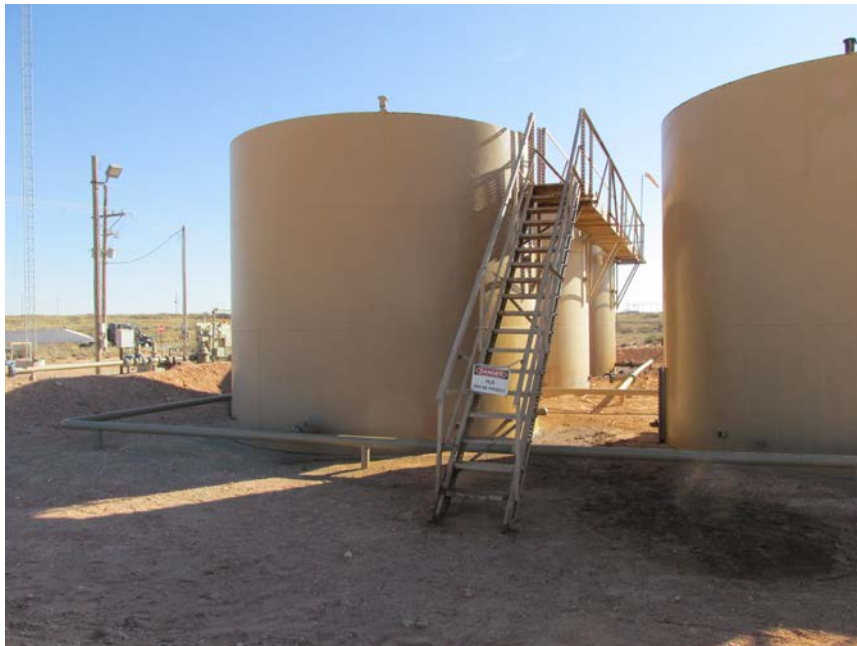
PHOTO 2: VIEW FACING NORTH EAST OF THE TANK BATTERY SHOWING PRODUCT SATURATED SOIL AROUND TWO CRUDE OIL TANKS
