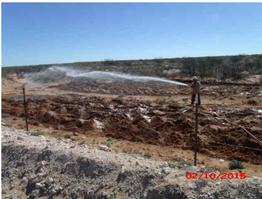
Photograph #7 – Micro-Blaze applied to remediation cells
