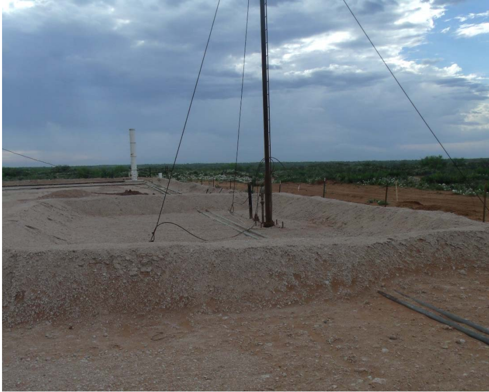
Photograph #11 – Pad area backfilled
