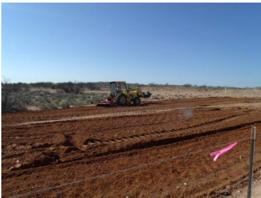
Photograph #8 – Tilling remediation cells
