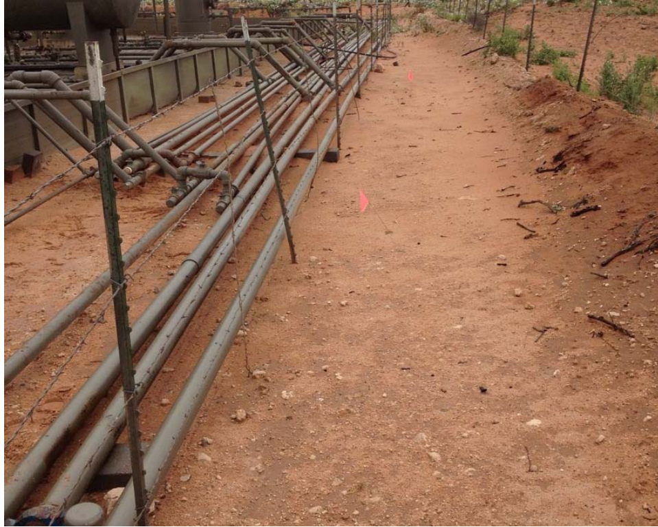
Photograph #13 – Pad area backfilled
