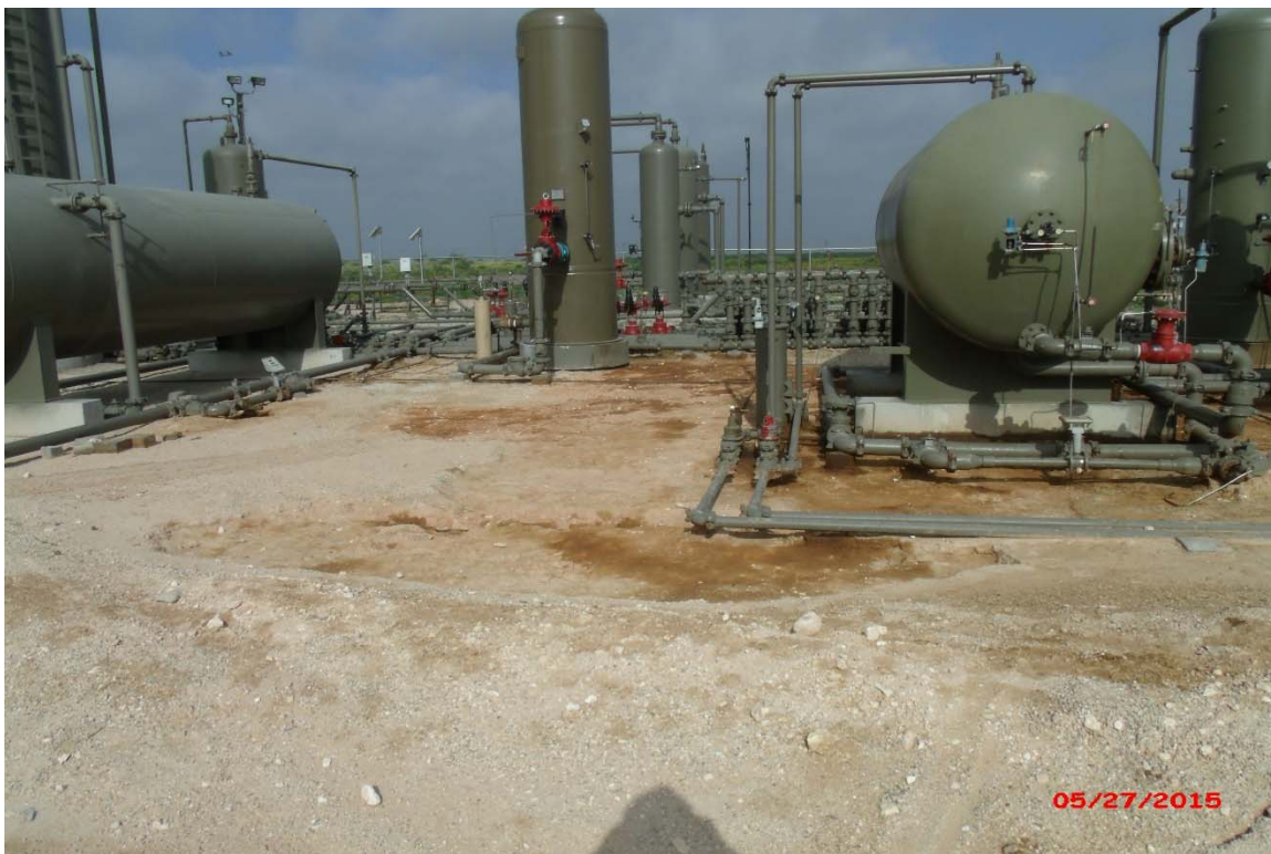
Photograph #3 – Release area excavated with Hydro-Vac
