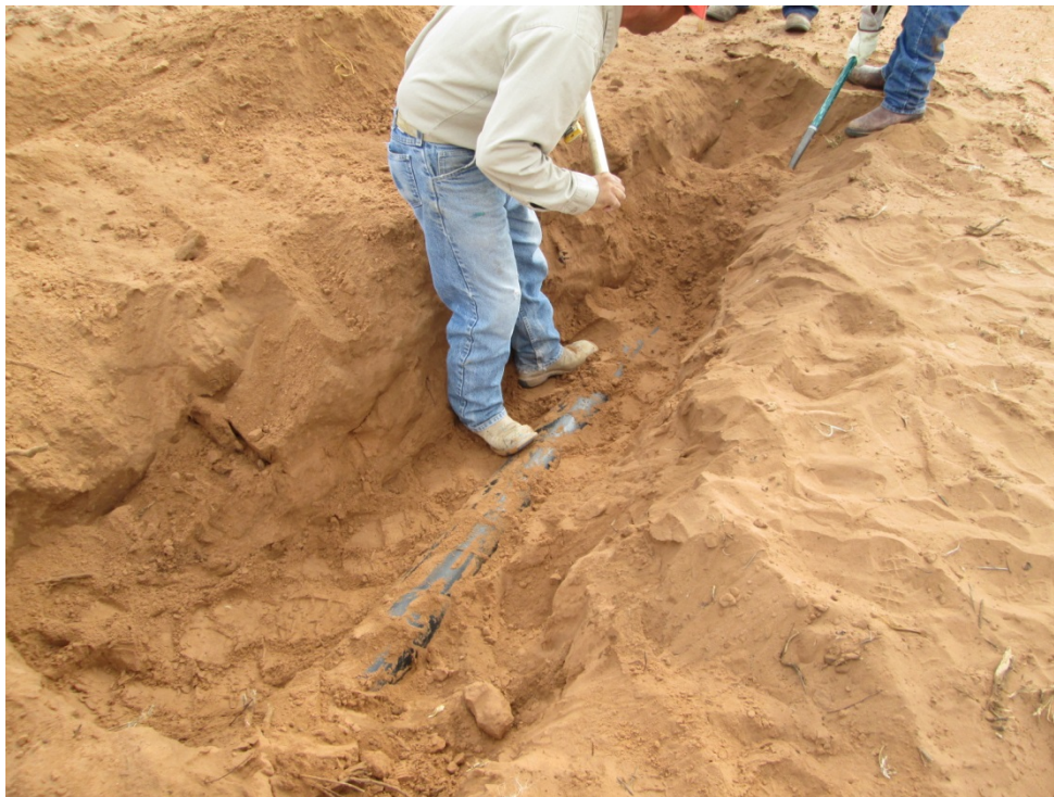
Photo 5 – August 5, 2014: Spotting of the pipeline.
