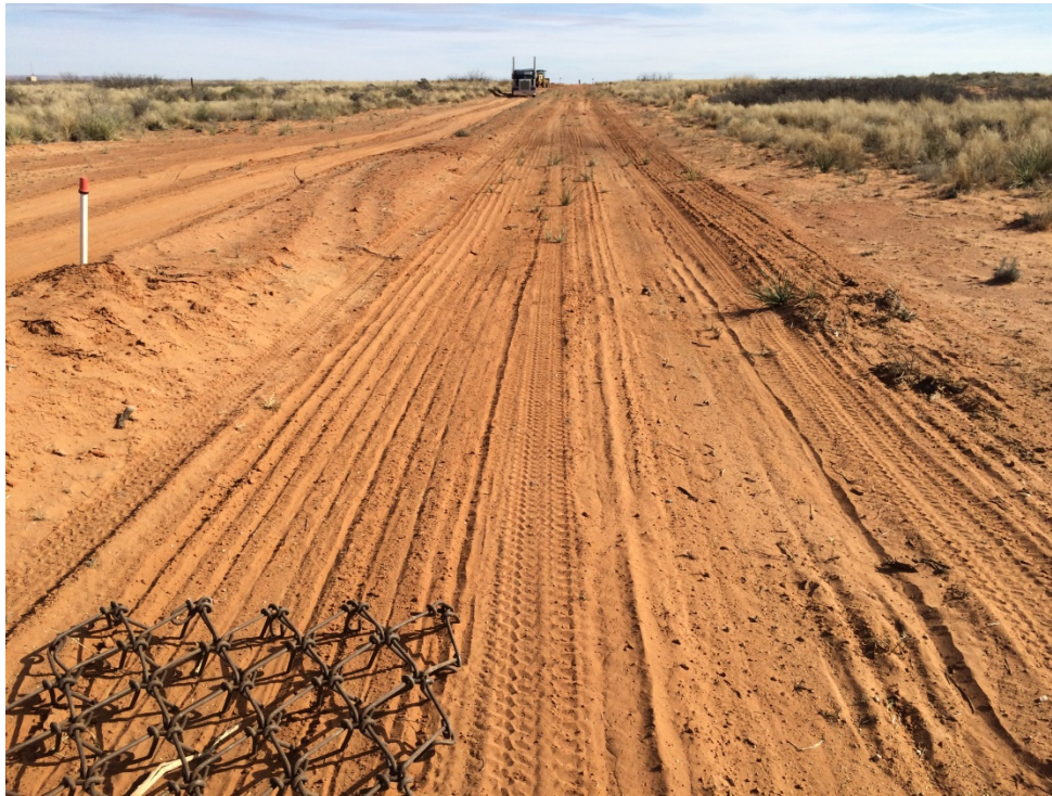
Photo 11 – December 16, 2014: Harrow used to till the BLM seed mix into the topsoil.
