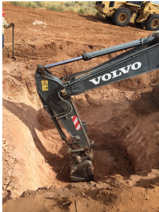
Photo 8 – August 26, 2014: Deepening of the excavation to 18 feet.
