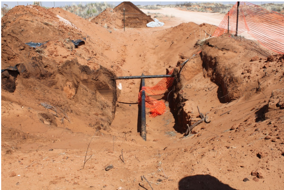
Photo 2 – March 26, 2014: looking north showing the emergency excavation around the Phillips 66 Pipeline (top) and HEP RJU South 4" Pipeline (bottom).
