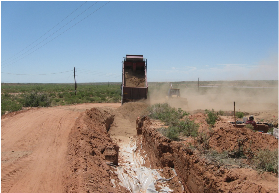
Photo No. 10: View to the west of backfilling operations along the access road of AOC No. 1, which would be surface completed with a caliche road-base.
