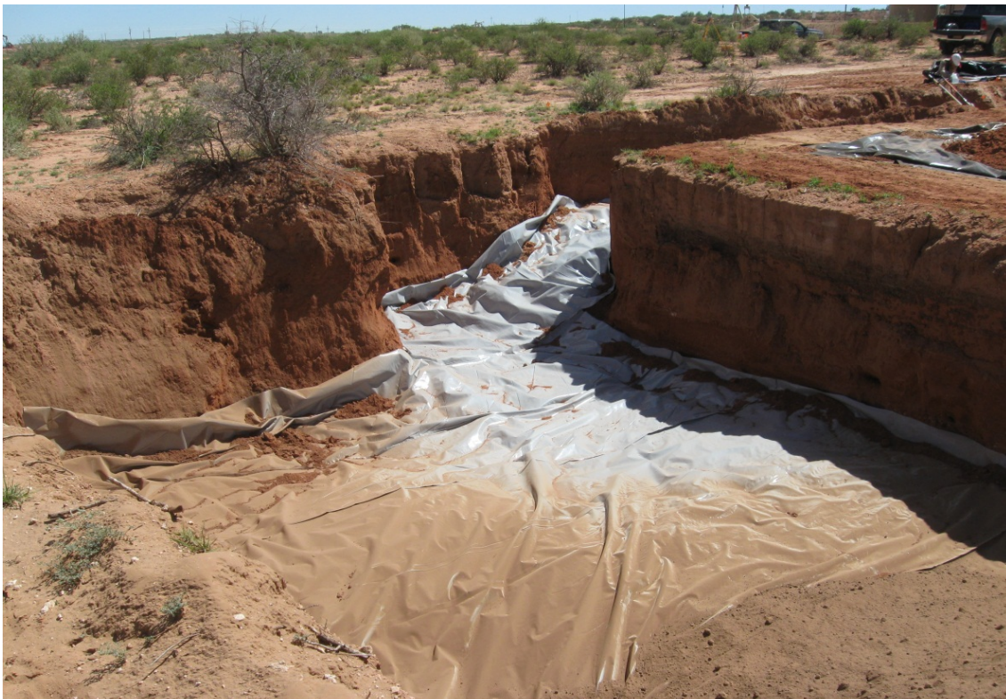
Photo No. 8: View to the north of the installed 20-mil high density polyethylene liner placed on along the western limits of AOC No. 1 at the 4-foot level of the excavation and a total depth of 8 ft-bgs.
