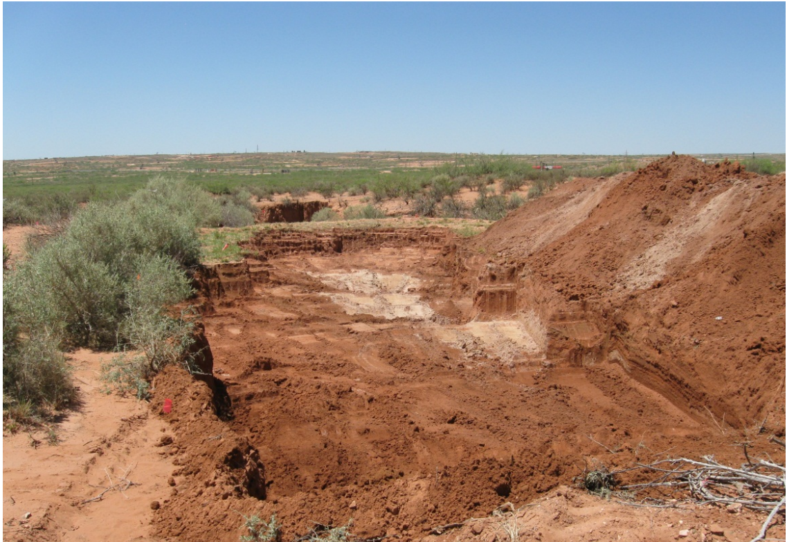
Photo No. 21: View to the north of the final limits of the AOC No. 3 soil excavation at 2ft-bgs.
