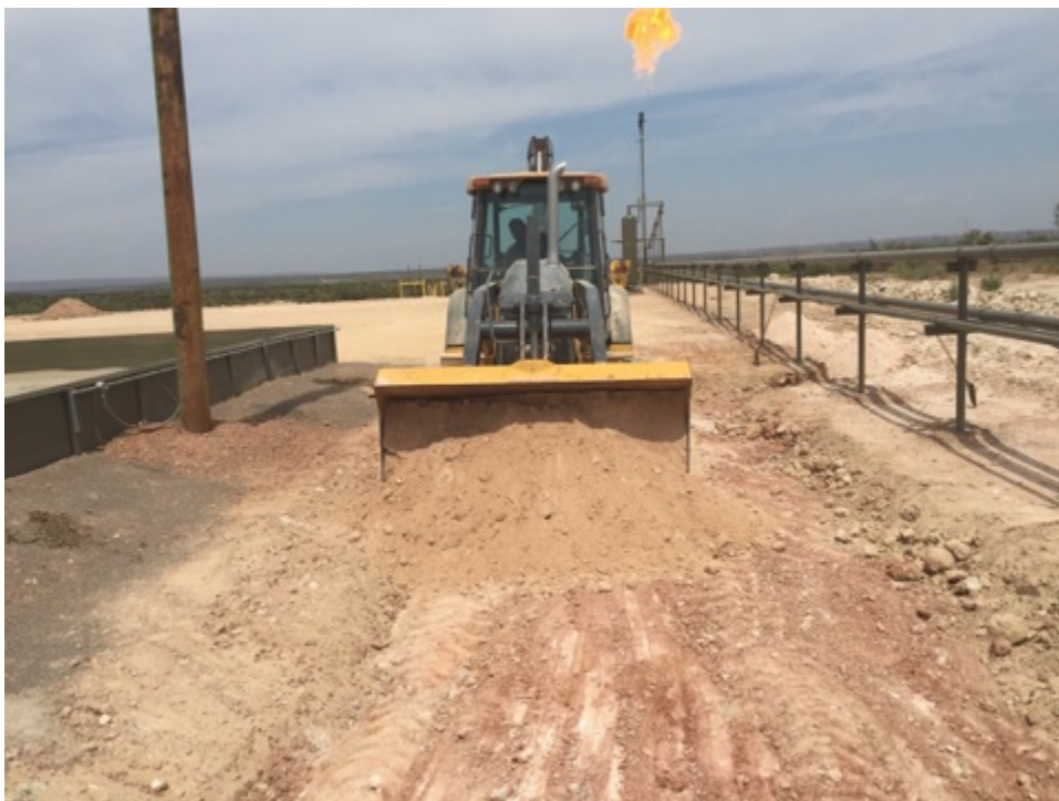
Backfilling excavated area with fresh caliche
