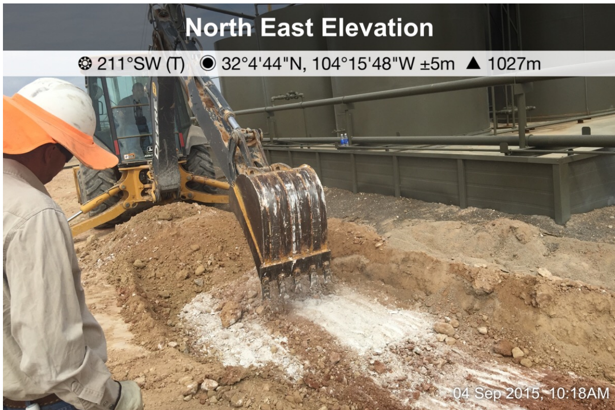
Digging to 1' bgs behind battery area
