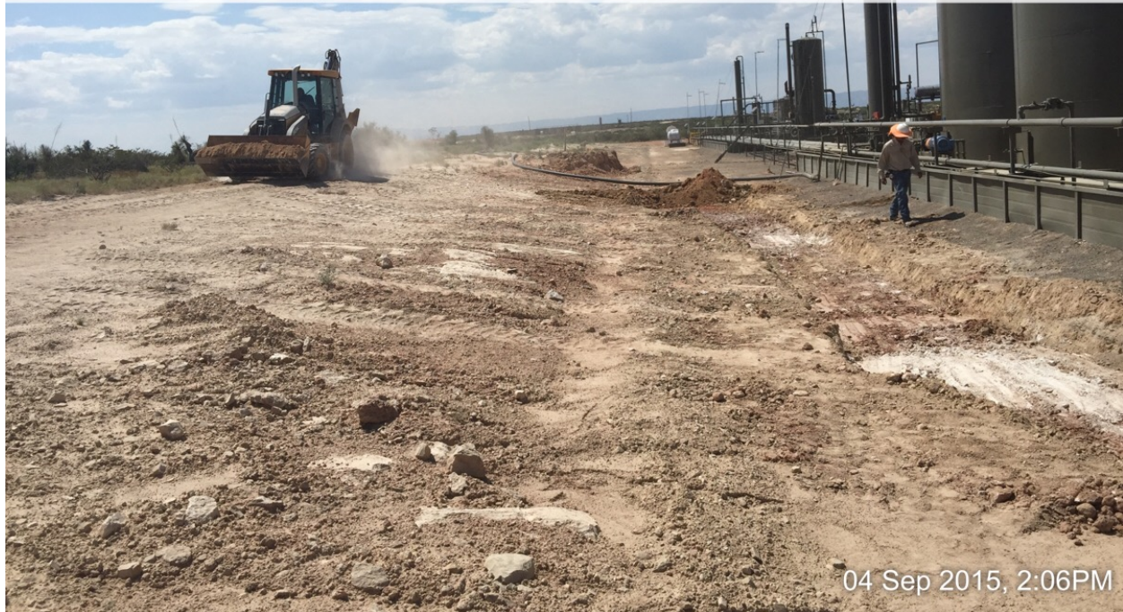
Hauling off contaminated soil after 1' excavation behind battery
