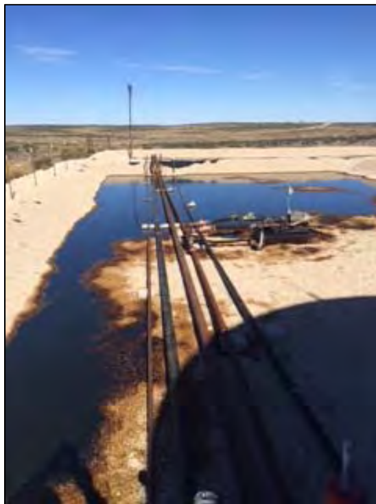
11/11/2015 Oil in secondary containment
