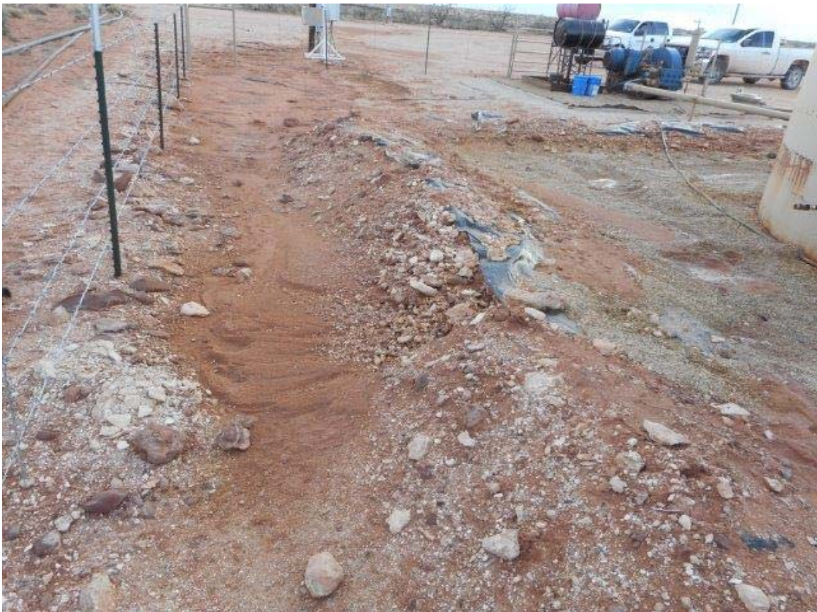
Viewing West: Natural slope and the tank berm channeled the flow westward
