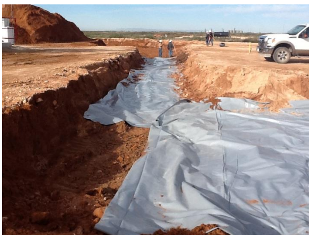
Liner Installation 10-23-15
