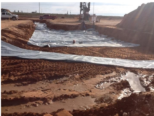
Liner Installation 10-23-15
