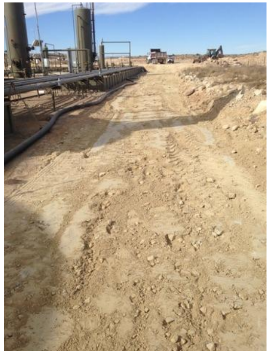
Spill area fully excavated and backfilled with fresh caliche, site completed
