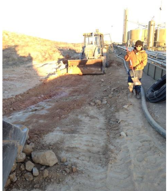
Excavating spill area behind battery
