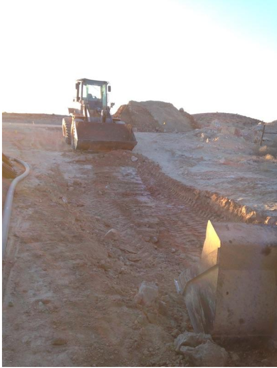
Excavating spill area behind battery
