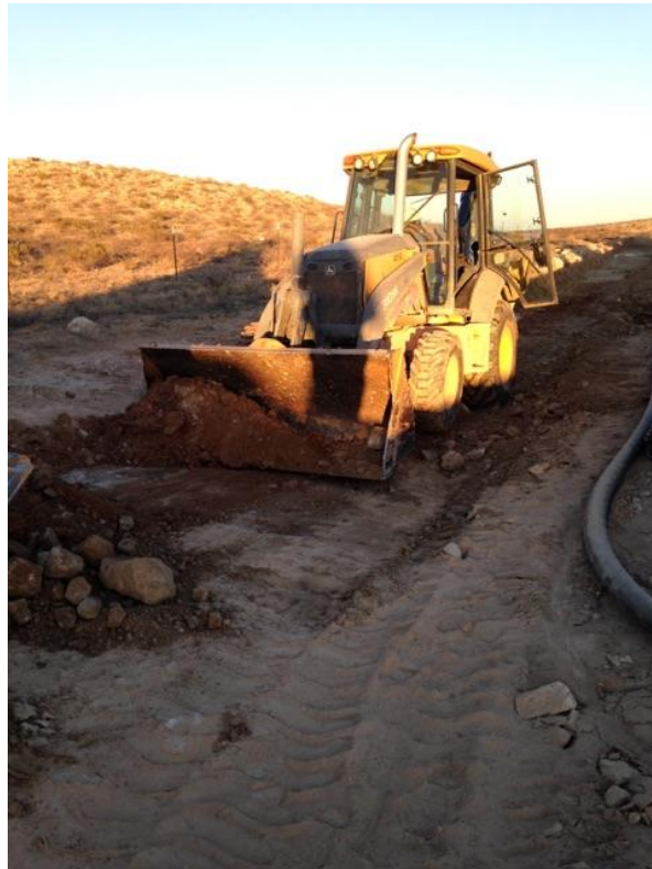
Excavating spill area behind battery
