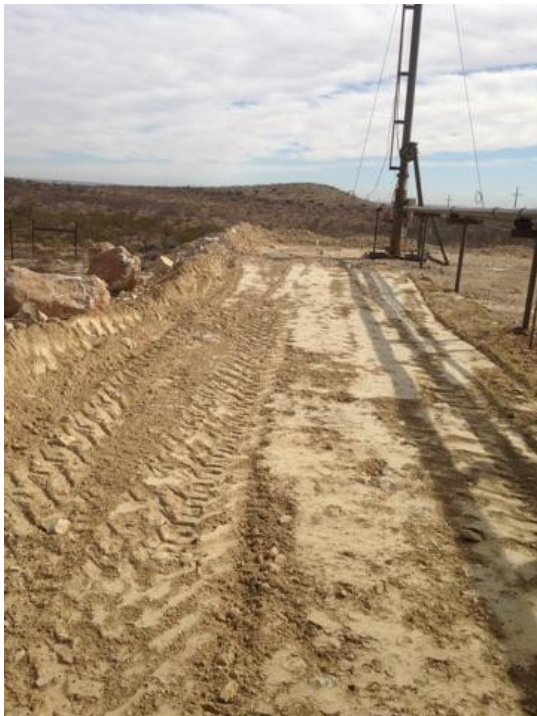
Spill area fully excavated and backfilled with fresh caliche, site completed
