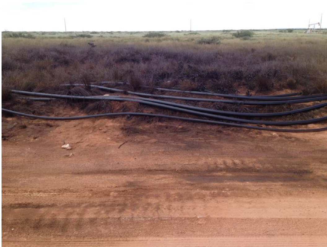
Leak #1 caused by vehicle exhaust
