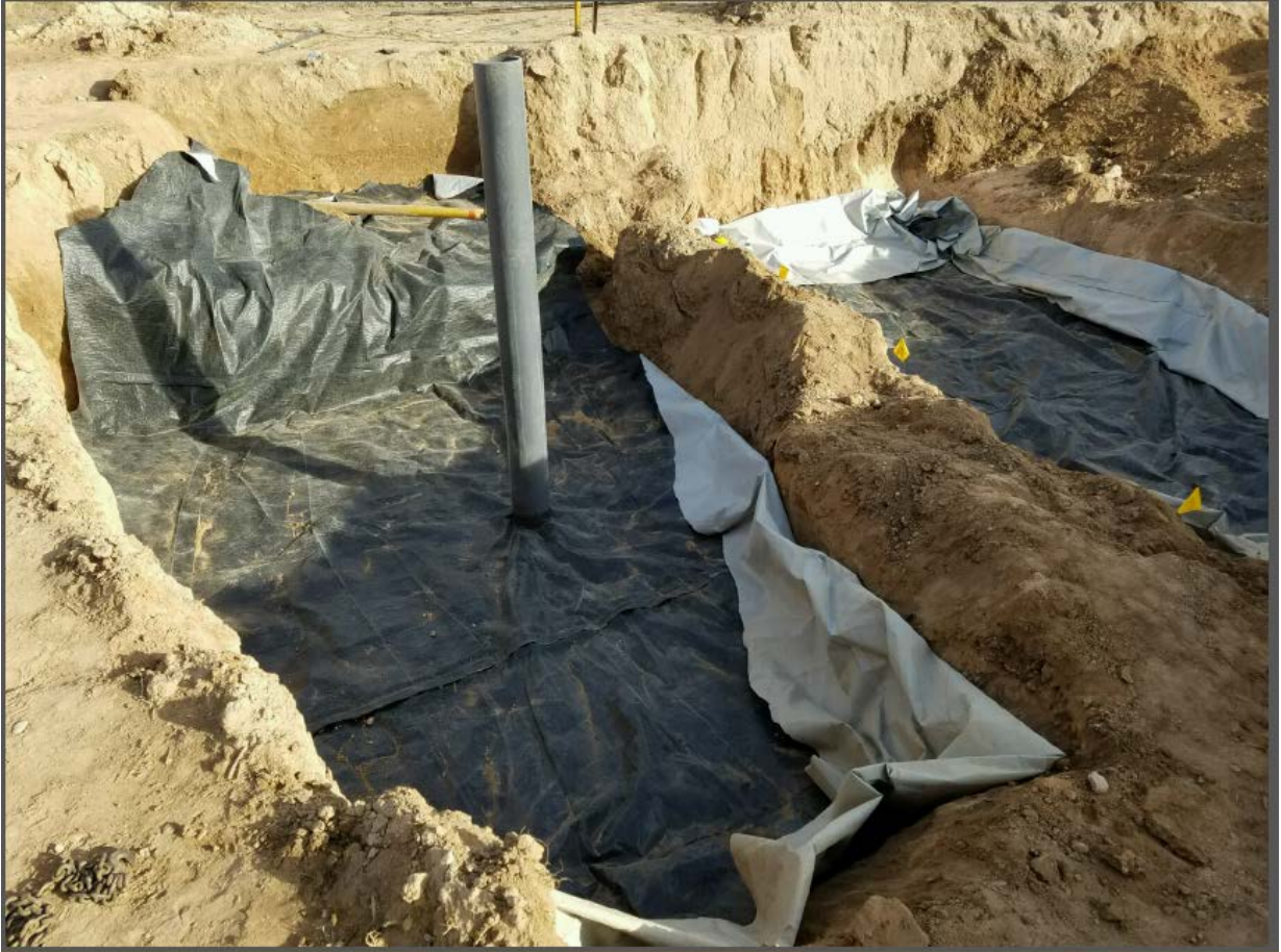
Photo for liner installed into bottom of excavated area.
