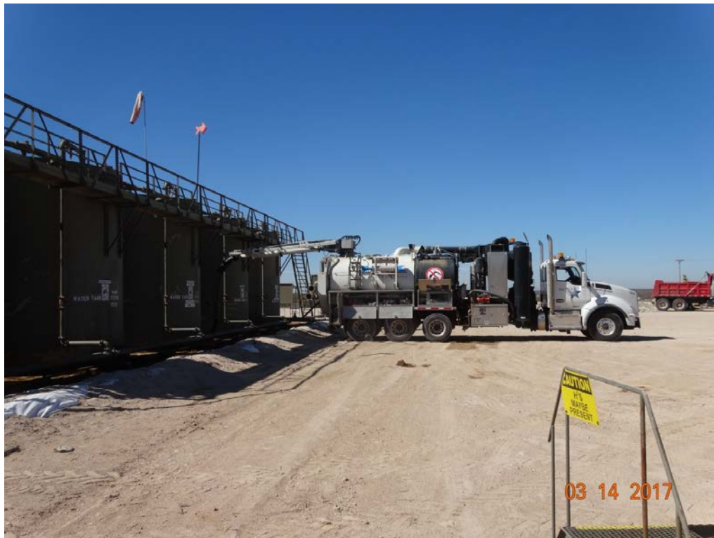
Hydrovac Truck Removing Gravel Viewing West
