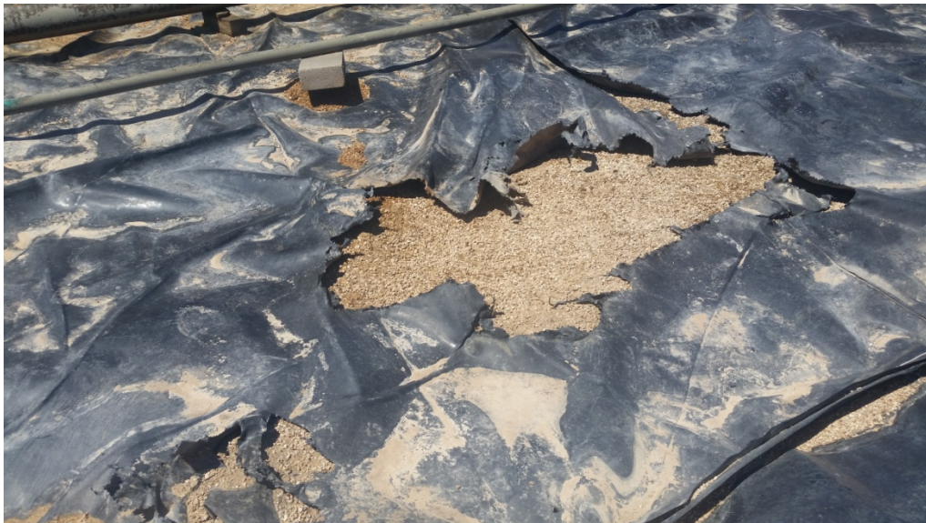
Break in Liner South of Tanks May 12, 2017
