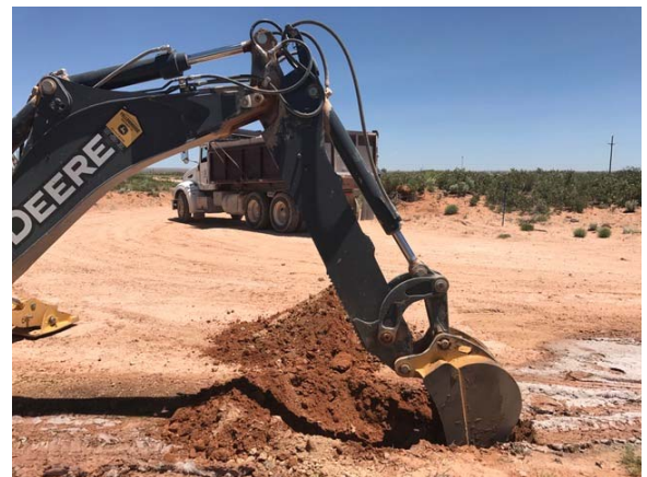
Excavating contaminated soil
