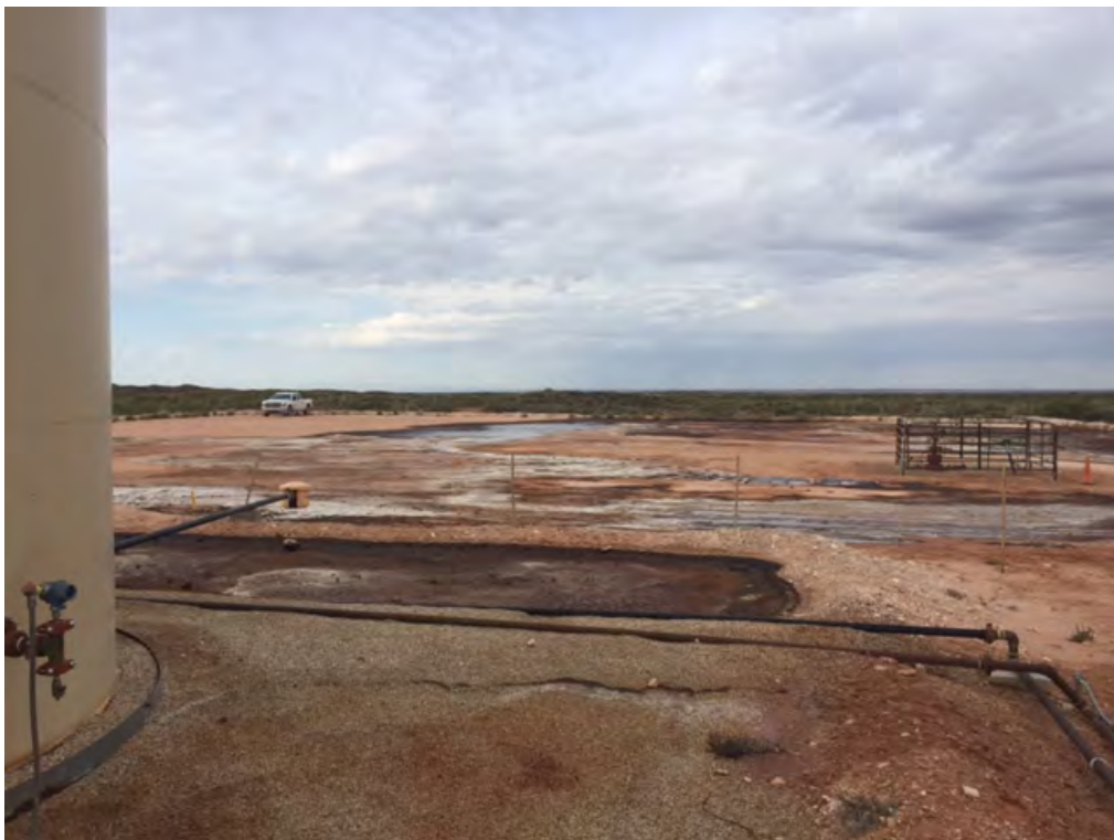
Lost Tank 33 Federal #2 SWD – Release (Looking West)
