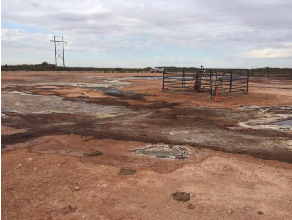
Lost Tank 33 Federal #2 SWD – Release (Looking Southwest)
