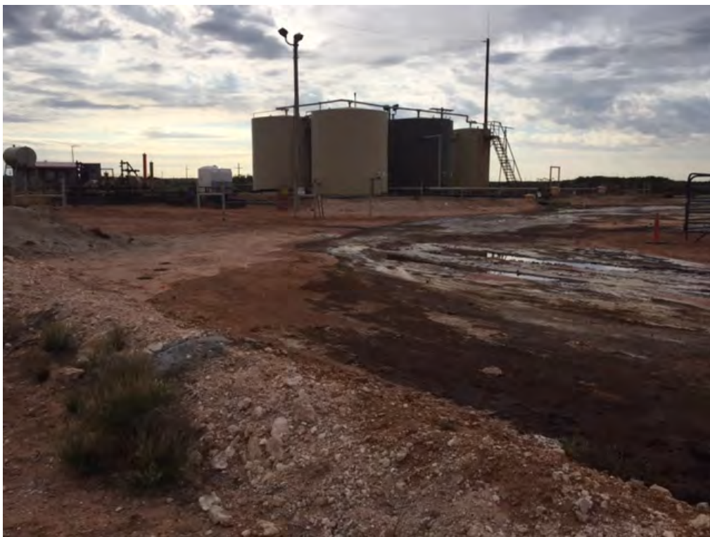
Lost Tank 33 Federal #2 SWD – Release (Looking Southeast)
