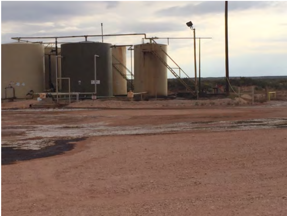
Lost Tank 33 Federal #2 SWD – Release (Looking East-Northeast)
