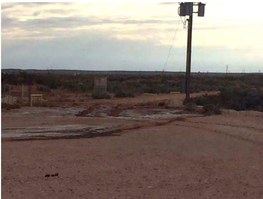
Lost Tank 33 Federal #2 SWD – Release (Looking East-Southeast)
