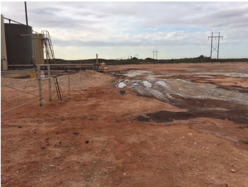
Lost Tank 33 Federal #2 SWD – Release (Looking South)
