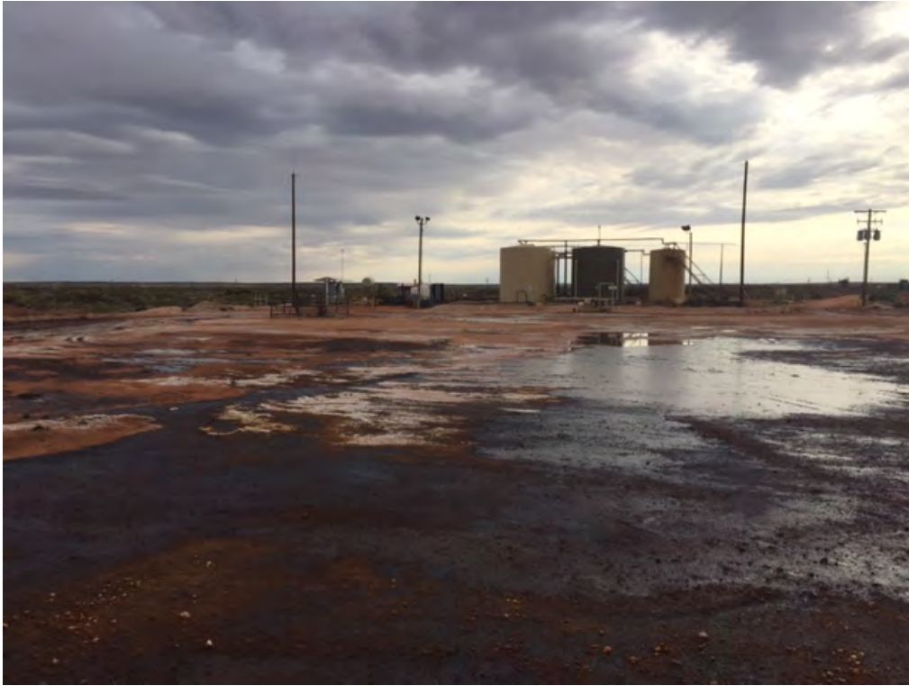
Lost Tank 33 Federal #2 SWD – Release (Looking East)
