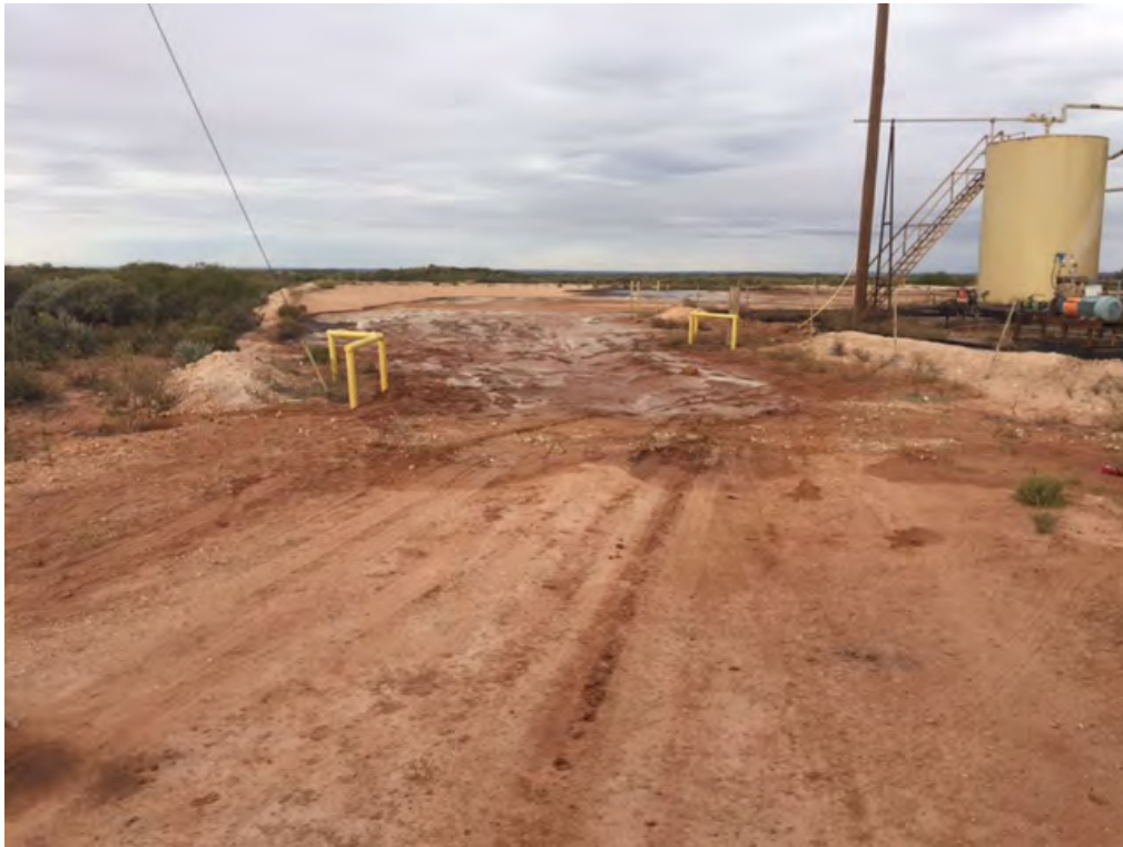
Lost Tank 33 Federal #2 SWD – Release (Looking West)
