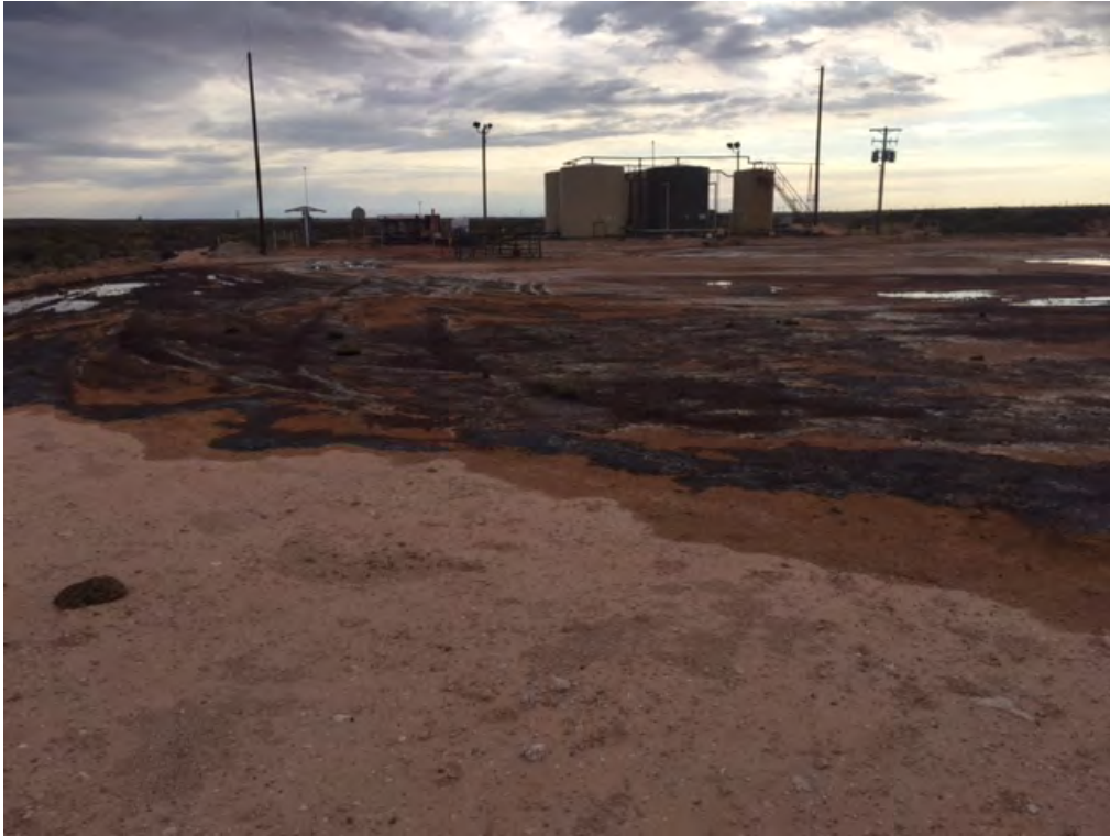
Lost Tank 33 Federal #2 SWD – Release (Looking East-Southeast)
