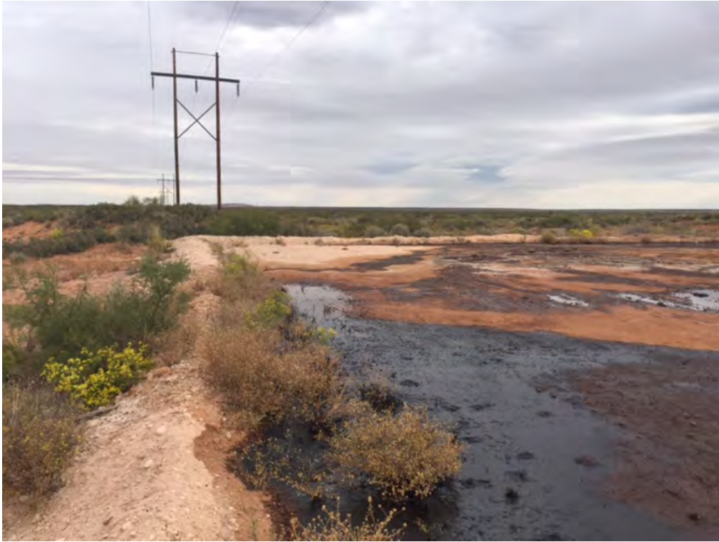
Lost Tank 33 Federal #2 SWD – Release (Looking North-Northeast)
