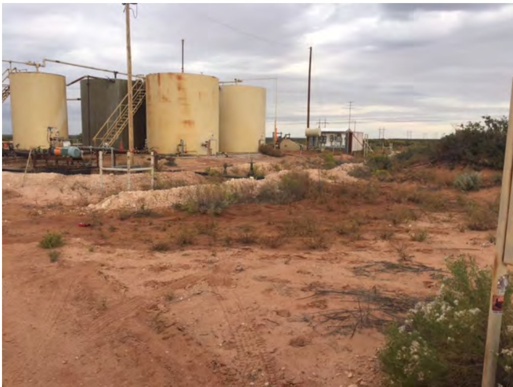
Lost Tank 33 Federal #2 SWD – Release (Looking North-Northwest)
