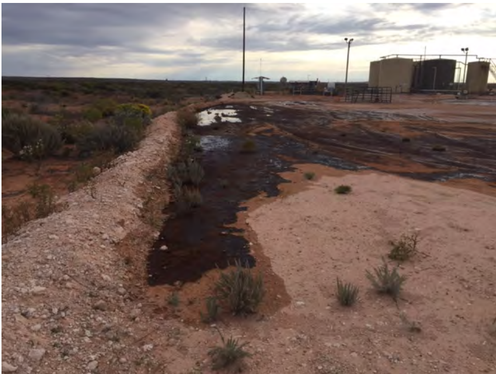
Lost Tank 33 Federal #2 SWD – Release (Looking East)
