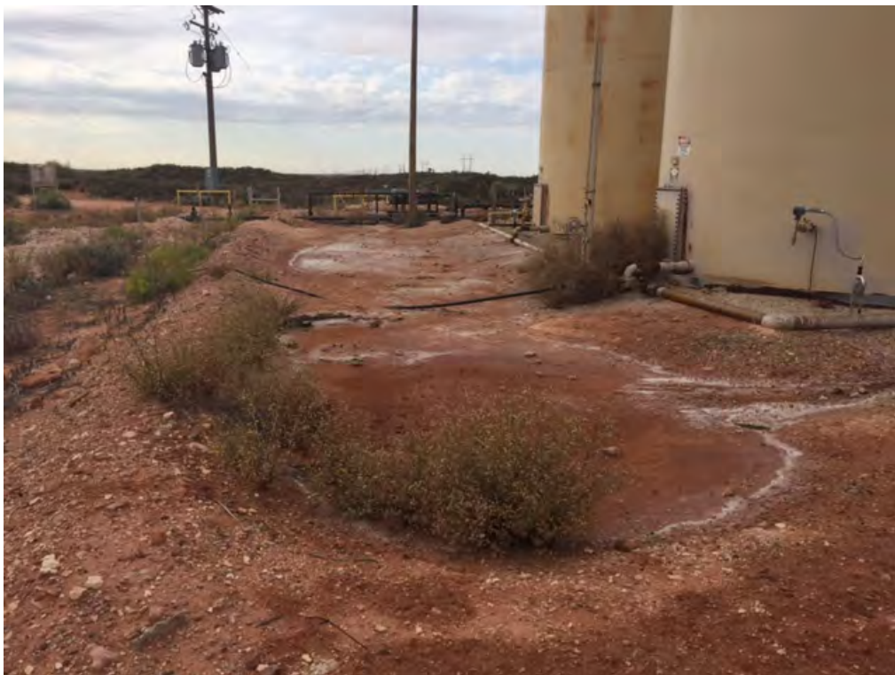
Lost Tank 33 Federal #2 SWD – Release (Looking South)
