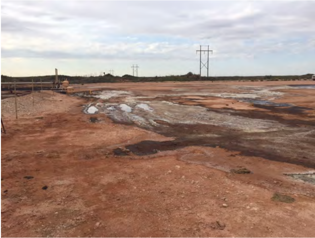
Lost Tank 33 Federal #2 SWD – Release (Looking South-Southwest)
