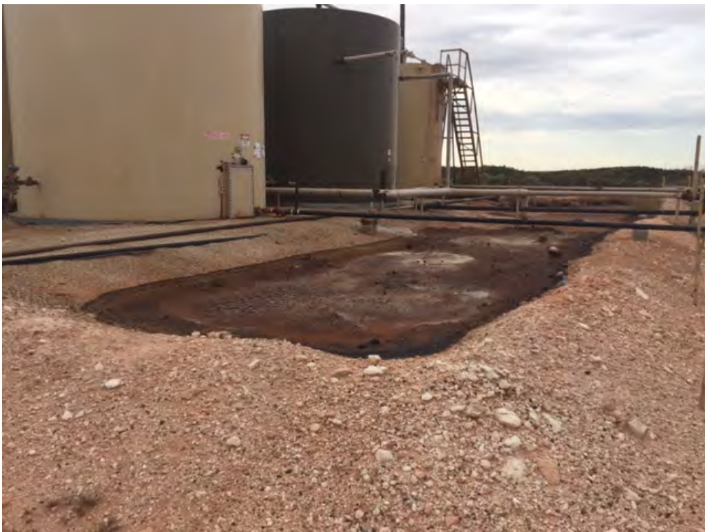
Lost Tank 33 Federal #2 SWD – Release (Looking South-Southeast)
