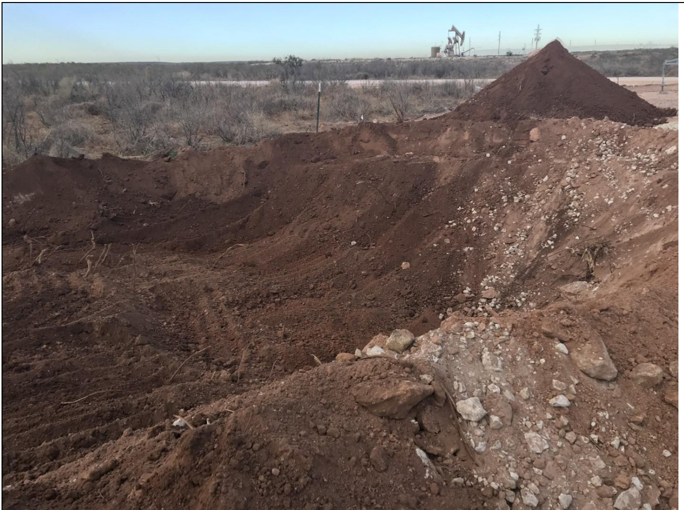
View of excavation facing southwest.
