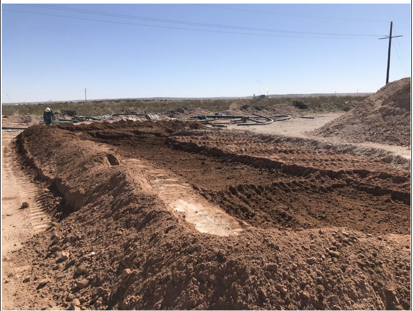
View of the excavation area southern boundary.
