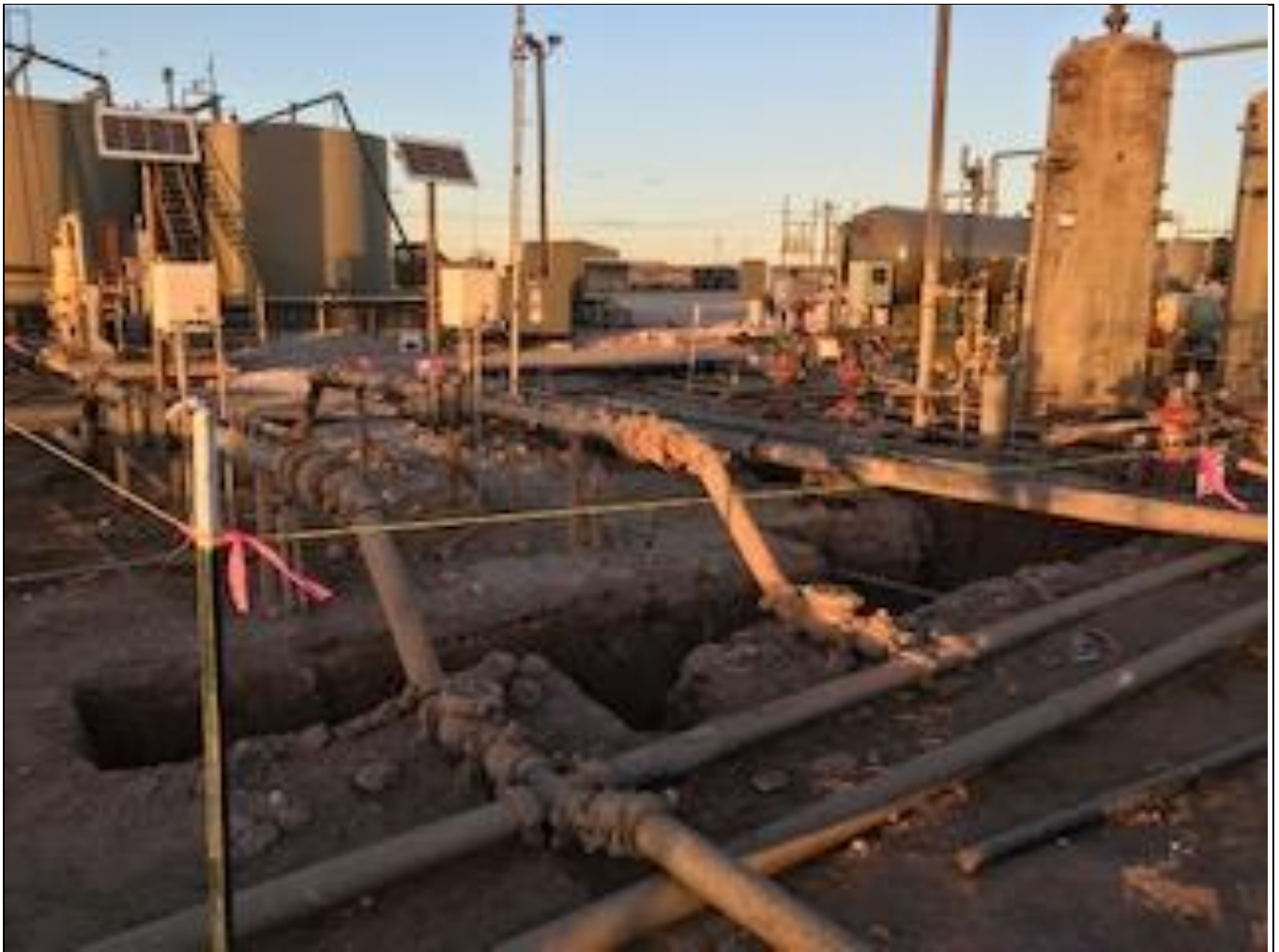
View northeast of excavation within both release areas (2RP-4399 and 2RP-5026)
