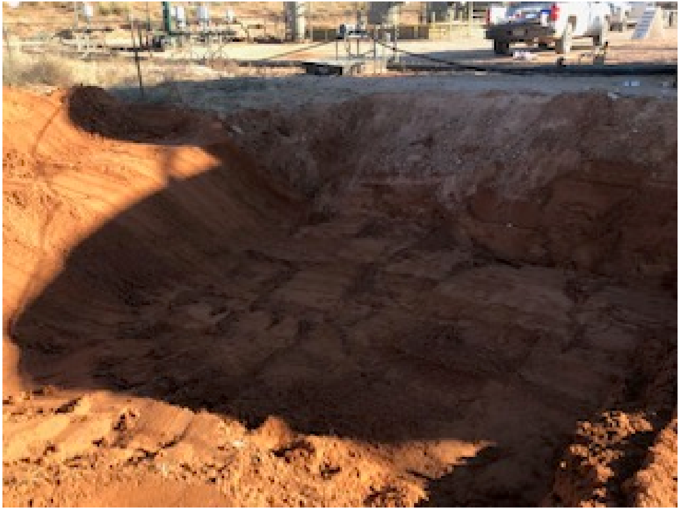
Southeast facing view of the excavation.
