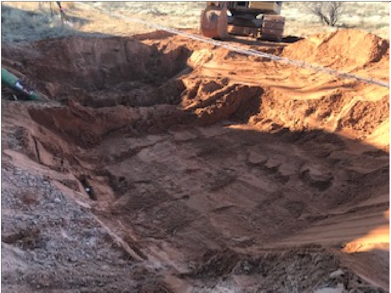
North facing view of the excavation.
