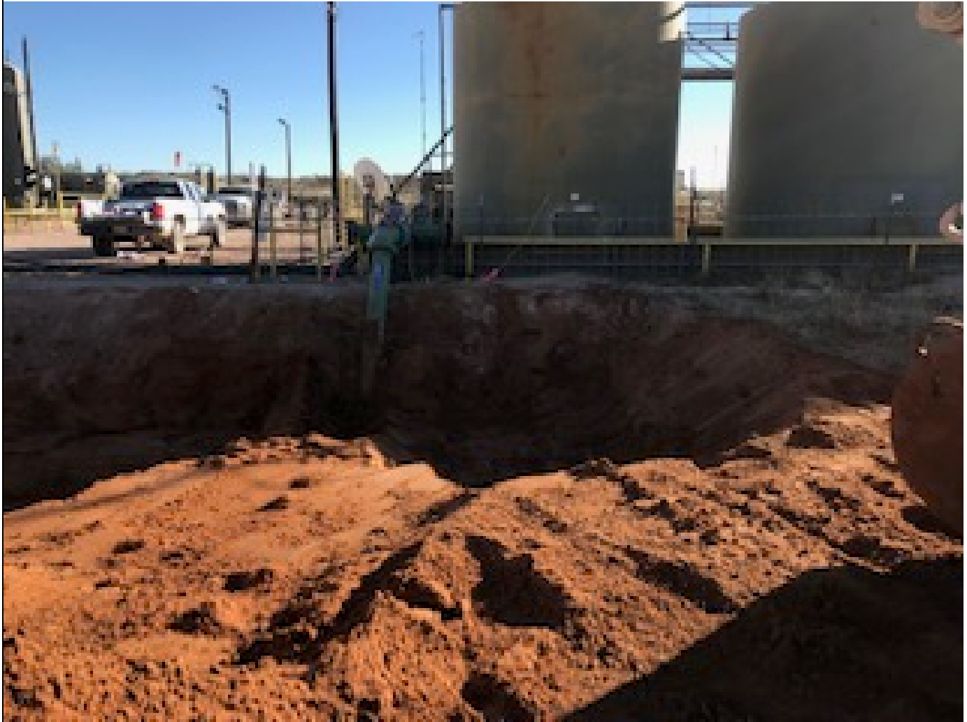
South facing view of the excavation.
