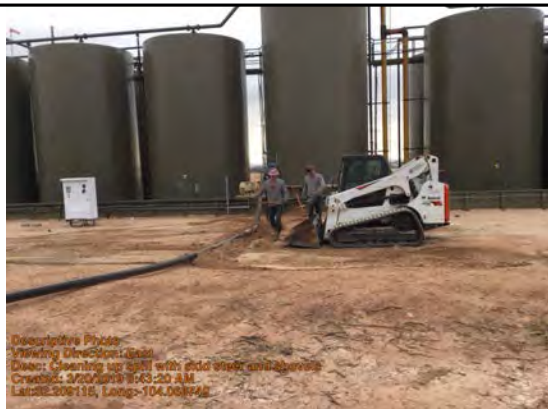
Cleaning up spill with skid steer and shovels
