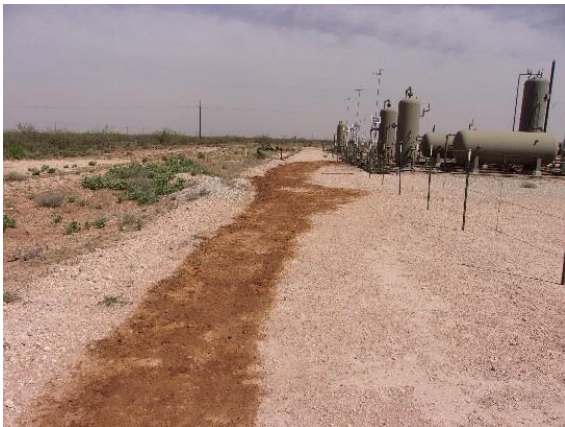
Impacted area facing North
