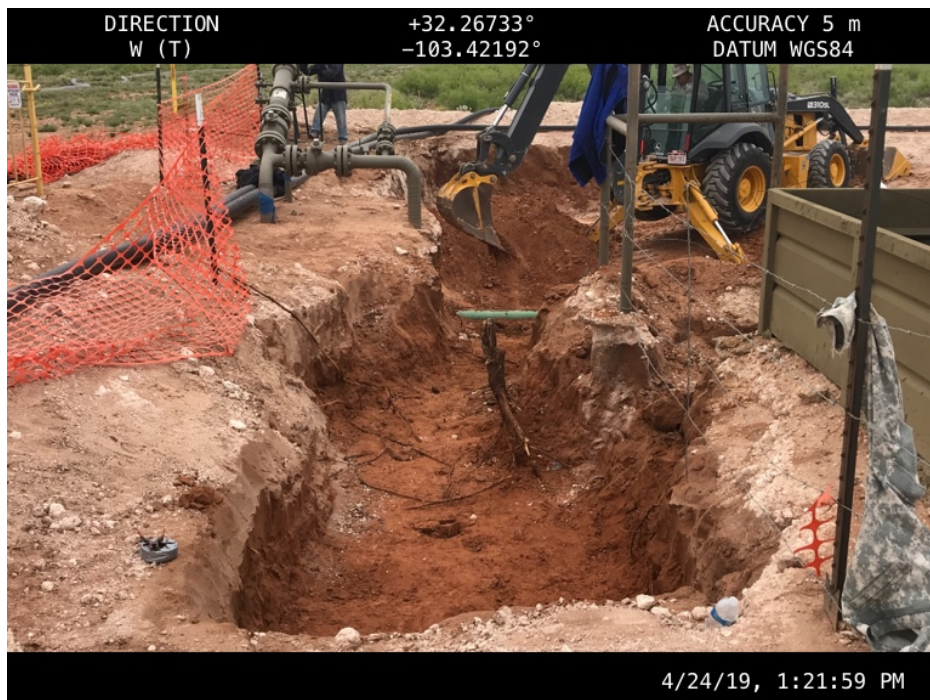
FL-2 Excavated from 1 ft. to 2 ft. bgs
