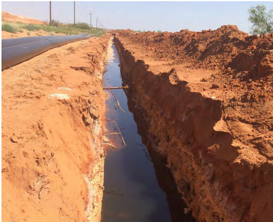
Figure 1: Produced water pooling in pipeline trench, viewing north. GPS: 32.4449083N, -103.6041028 W. Date/Time: 2019-08-01 10:18:38.
