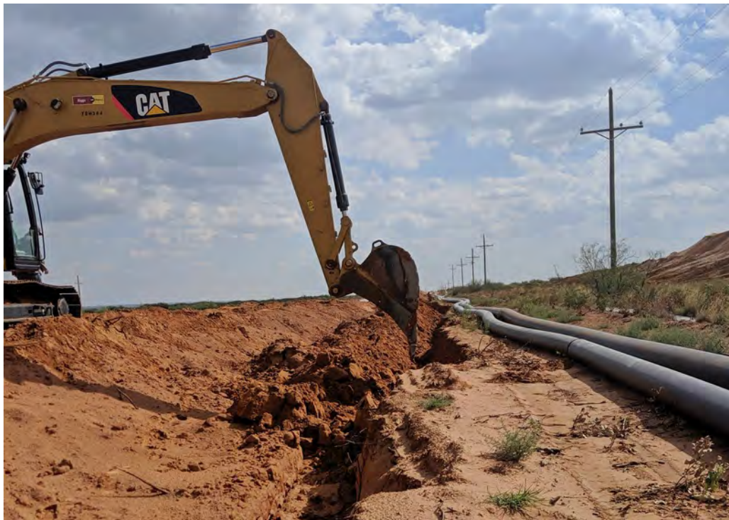
Figure 3: Excavation of the release within the pipeline trench. Photograph is viewing south from sample point T-02 (S-09). GPS: 32.4470472 N, -103.6041028 W. Time/Date: 2019-09-16 15:13:13
