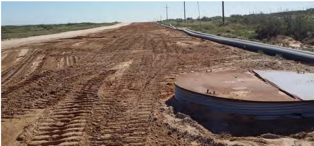
Figure 4: Final backfill and reclamation of pipeline-right-of-way. Photograph viewing south from the Source area. Date/Time: 2019-10-17 14:07:52. GPS: 32.4459915 N, -103.6039734 W.
