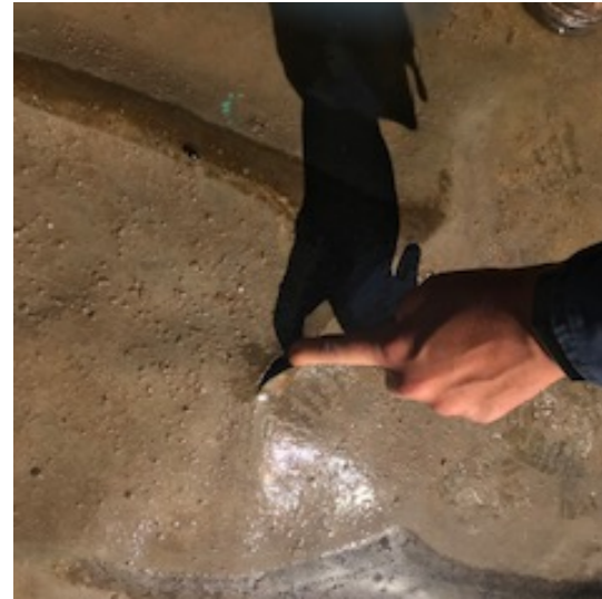
Photograph 2: Liner tear.
