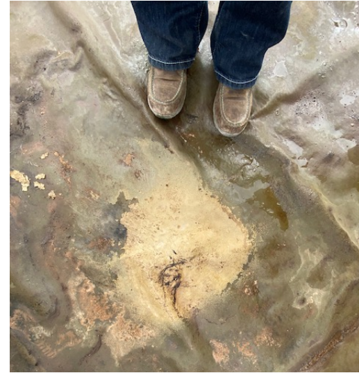
Photograph 2: Second liner tear repair
