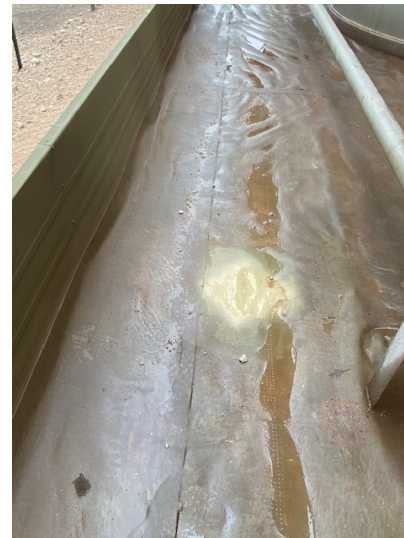
Photograph 4: Completed liner repair.
