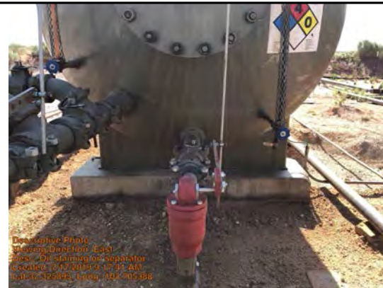
Oil staining on separator 6-2
