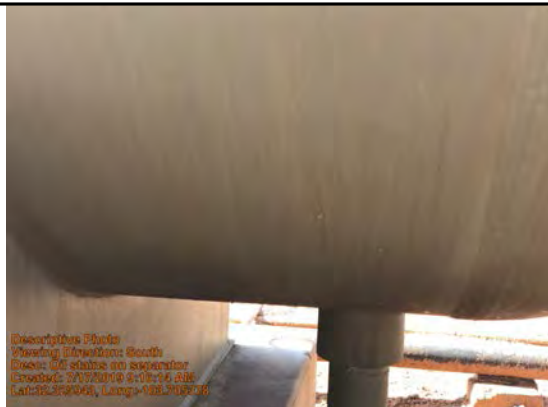
Oil stains on separator 6-2
