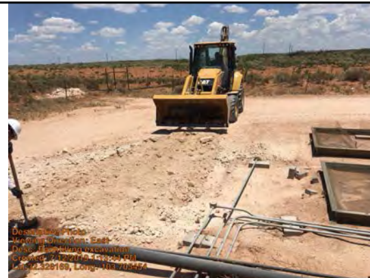
Backfilling excavation
