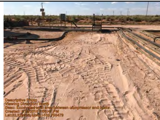
Excavated spill area between compressor and tanks
