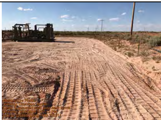
Excavated spill area near fence
