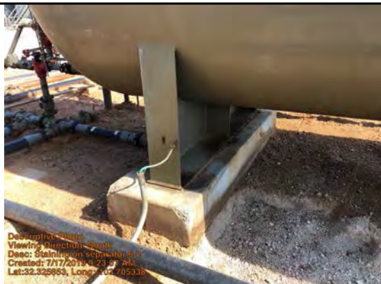
Staining on separator 6-2
