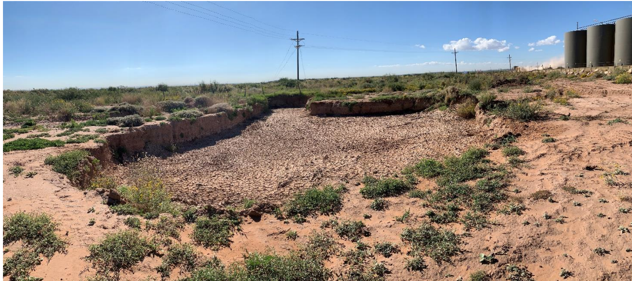
Photo 5: 4' Excavated area around BH2 & BH3.
