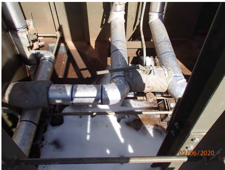
View of snow and water inside the secondary containment.
