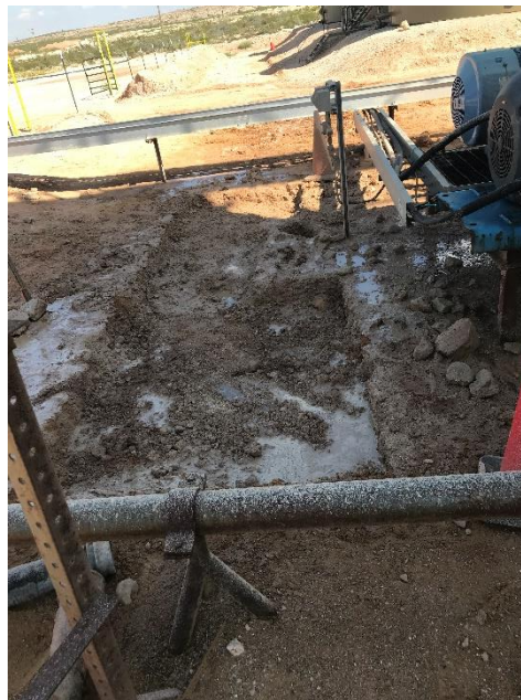
View of the excavation down to the exposed clay liner.
