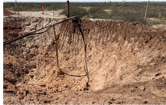
Photograph 4: View of excavation beneath surface flowline.
