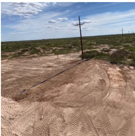
Photograph 5: View of final backfill.
