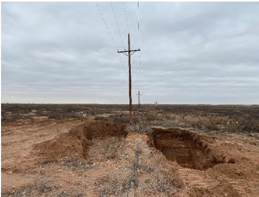
Photograph 3: View of initial two excavations on either side of the surface flowline.
