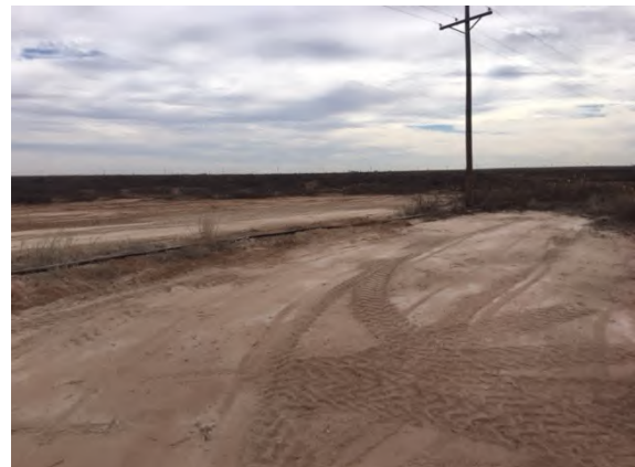
Photograph 6: View of final backfill.
