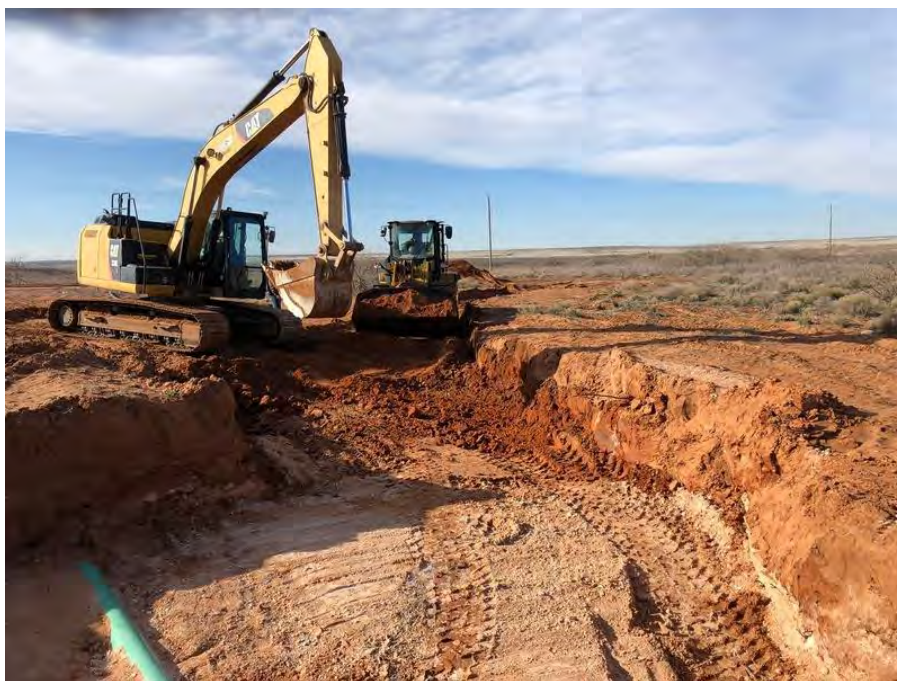
Figure 4: Excavation of bases and wall until electrical conductivity (EC) <0.2 dS/m. Date 02/13/2020. GPS: 32.4198528 N, 103.6048194 W
