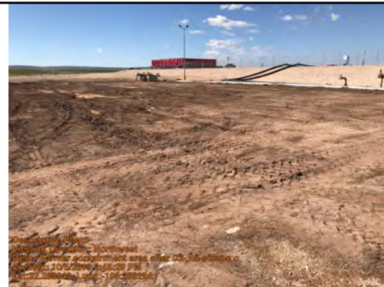
Former containment area after 0.5' scrape off
