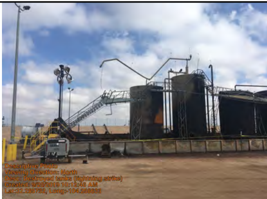
Destroyed tanks (lightning strike)
