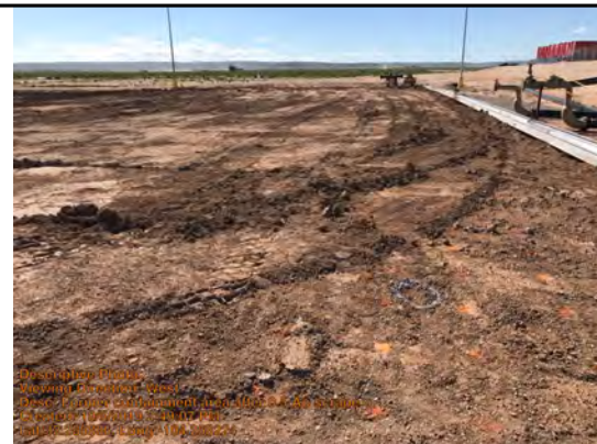
Former containment area after 0.5' scrape off
