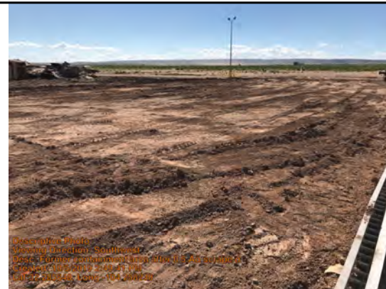
Former containment area after 0.5' scrape off
