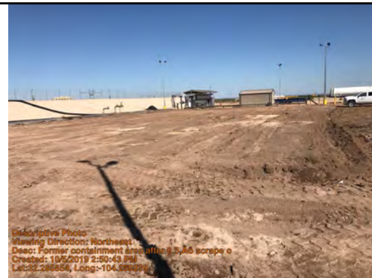
Former containment area after 0.5' scrape off
