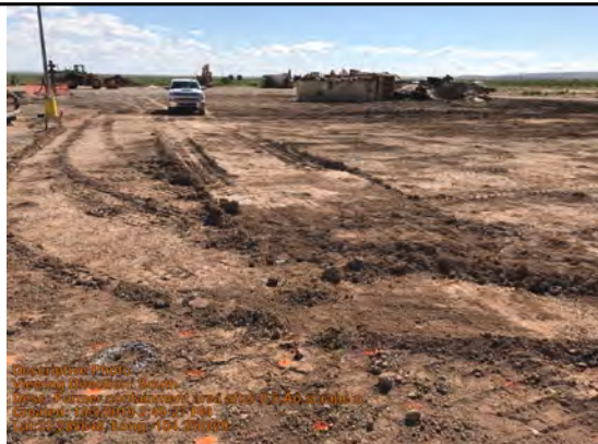
Former containment area after 0.5' scrape off
