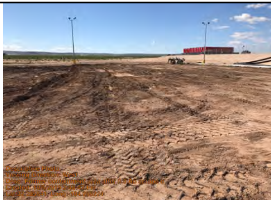
Former containment area after 0.5' scrape off
