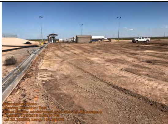
Former containment area after 0.5' scrape off
