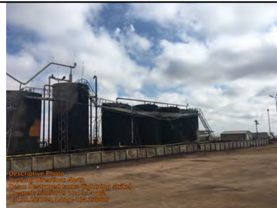
Destroyed tanks (lightning strike)
