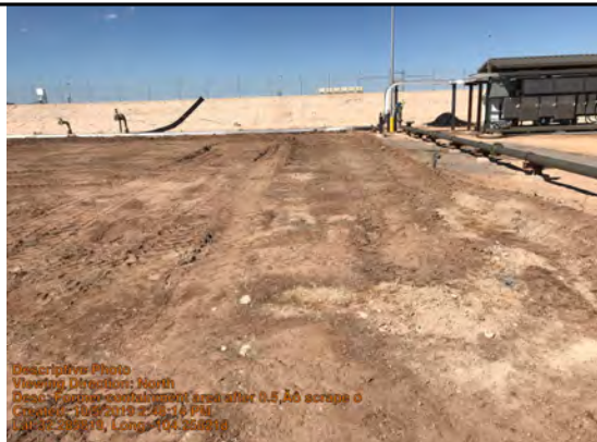
Former containment area after 0.5' scrape off
