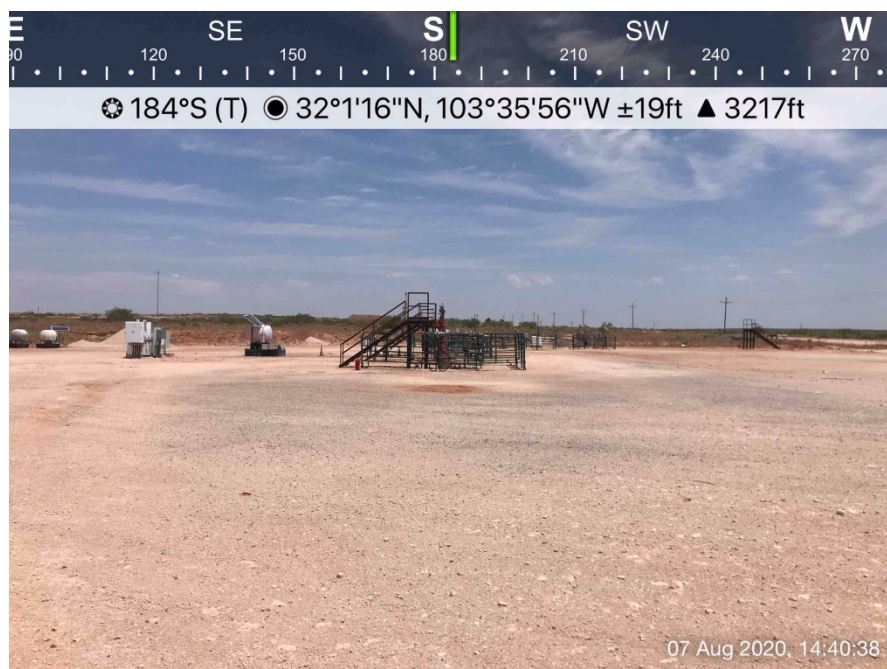
Spill area viewing south
