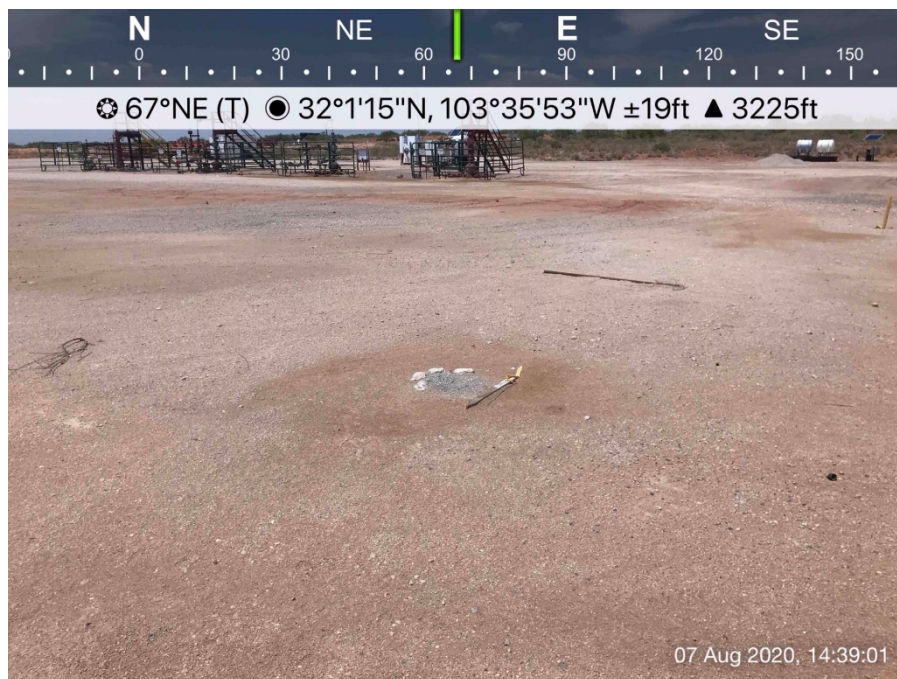
Spill area and S-5 viewing Northeast/East
