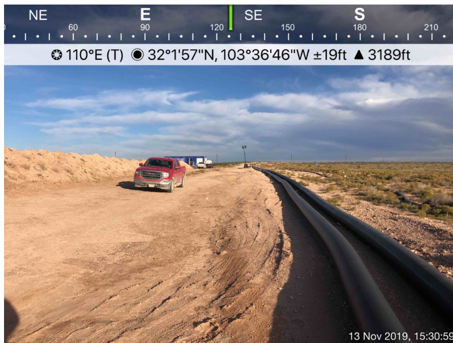
Spill area viewing southeast
